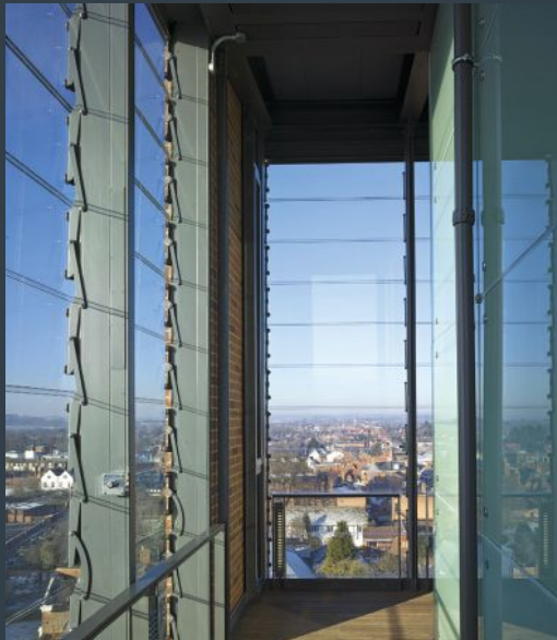
Louvered Facade Ventilators
