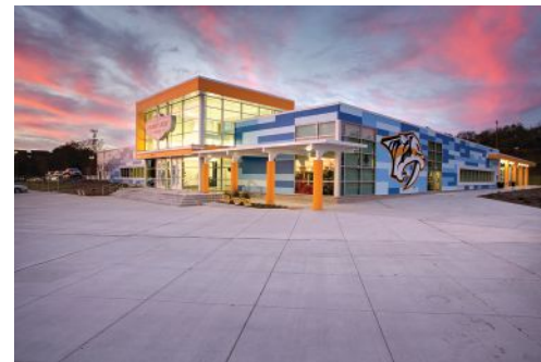
A successful wall design provides multiple pathways for drainage and doesn't allow the water to build up in the wall system. Photo courtesy of Nichiha
