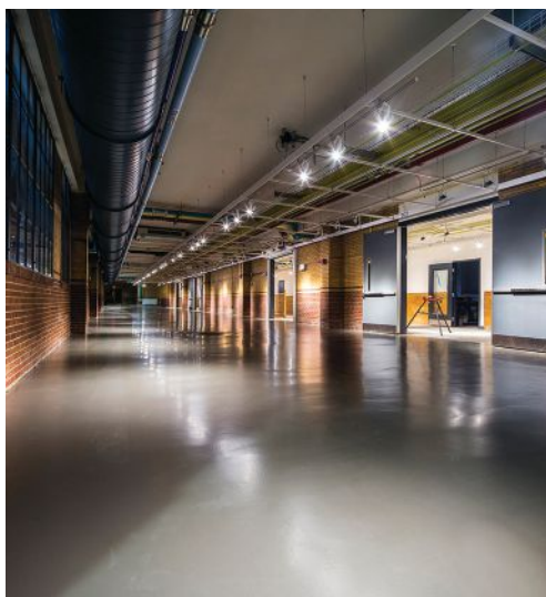
Recent developments of polyaspartic and waterborne polyurethane coatings and sealers address many of the desired attributes sought by the formulator, contractor and owner such as chemical and stain resistance, low odor, long term performance, ease of use and concrete penetration. Photo Courtesy of Bayer MaterialScience
