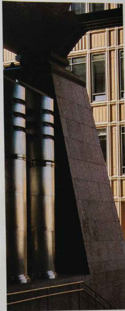
Struts (left) provide lateral support to the exterior frame by tying it back to interior girders. At the base of each arch the major structural elements join at a node (bottom left and below). Loads are then transferred to buttressed piers (above).
