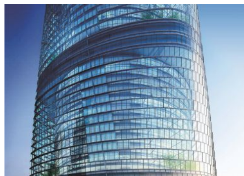
The curtain wall consists of more than 20,000 interior and exterior panels with more than 7,000 unique shapes. © Gensler
