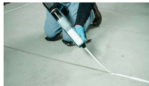
Due to increased demand for higher durability concrete sealers, waterborne polyurethane technology is now considered a replacement for traditional acrylic stainguard products. Photo Courtesy of Bayer MaterialScience
