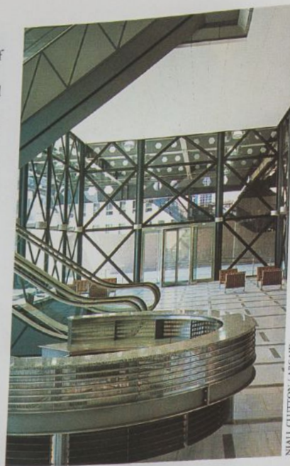
The lobby and elevators are enclosed in glass to create a sense of transparency (above), in contrast to the solid structural members. Interior arches are partially revealed in two
