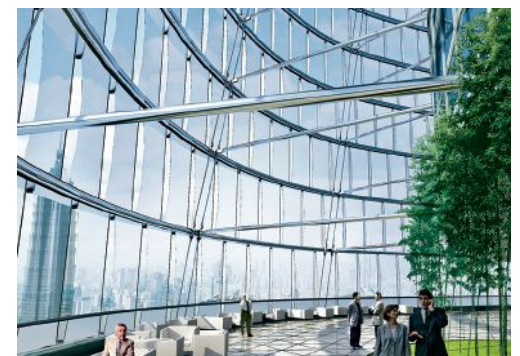
The building skin is suspended from above on huge cantilevered trusses that are stabilized by hoop rings and struts. © Gensler
