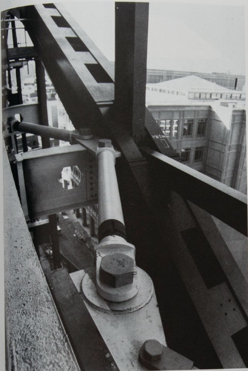
Struts (left) provide lateral support to the exterior frame by tying it back to interior girders. At the base of each arch the major structural elements join at a node (bottom left and below). Loads are then transferred to buttressed piers (above).
