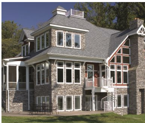
Bluff stone profile with dry stack grout gives the appearance that this home was built on a solid stone foundation. Photo courtesy of Eldorado Stone
