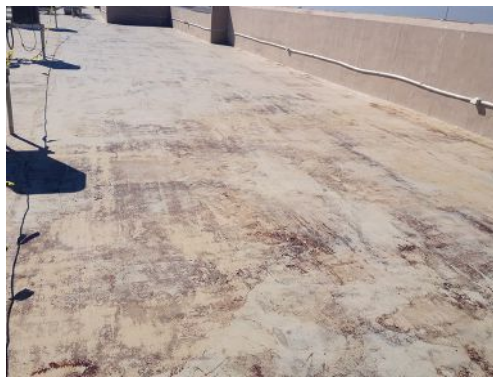
Liquid-applied coatings can be installed over virtually any type of existing roof substrate.
