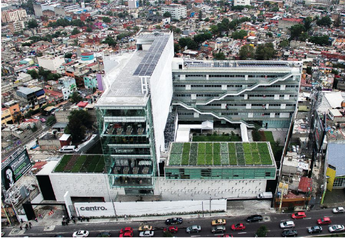
Aerial view from the northwest
