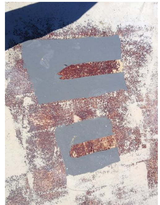
Primers can be used to darken substrates to reduce small amounts of residual moisture, as the darker surface will absorb more heat and dry faster.
