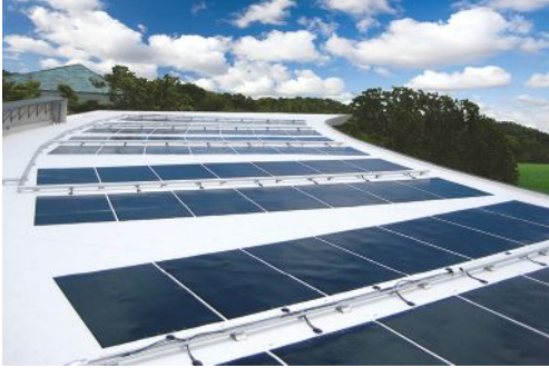
Figure 4 Flexible and flat, modern solar modules can help increase overall solar collection capacity while not interfering with the roof aesthetics.
