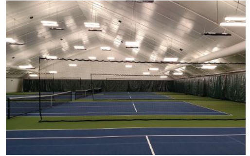
Figure 4 Oklahoma City Tennis Center: Indoor tennis courts and an LED lighting system.
