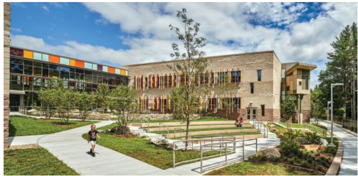
One of the courtyards behind the school
