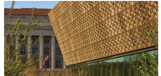
Each panel that was custom cast was finished with five different coating layers, each a different color of the coating, to achieve the exact bronze shade desired by the design team. Photo credit: Alan Karchmer
