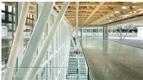
The Aspen Art Museum features an iconic, composite geometric screen that drapes the museum's bright glass and white metal exterior on two sides. The curtainwall, window, sliding door and skylight systems were finished with 70 percent PVDF coatings. Photo Credit: Derek Skalko
