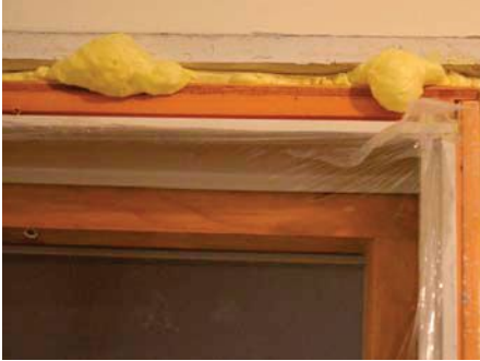
Spray foam flows, expands, seals, and hardens. As a result, it's ideal for insulating small and oddly-shaped openings.
