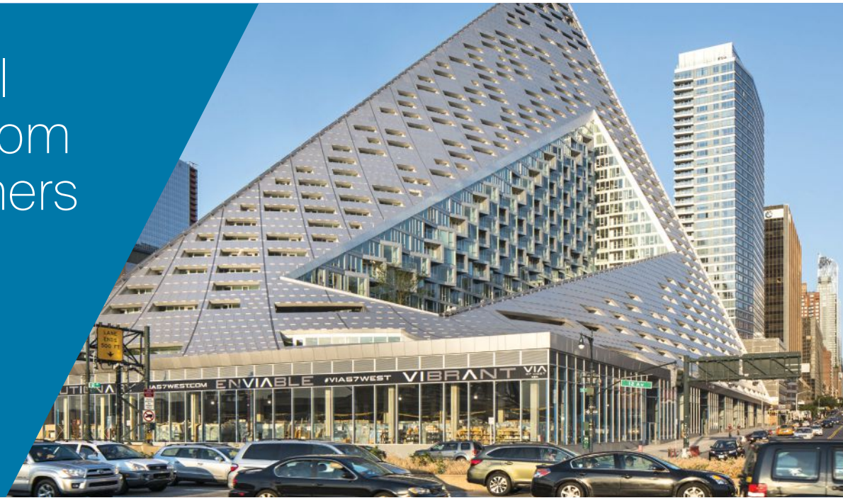
Via 57 West • New York, NY • Duranar Sunstorm Coatings
