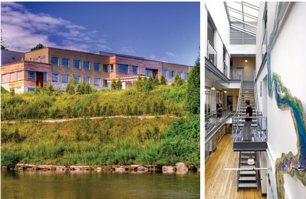
Enermodal Engineering Headquarters, Kitchener, Ontario. Photo courtesy of Nudura and Enermodel Engineering.
