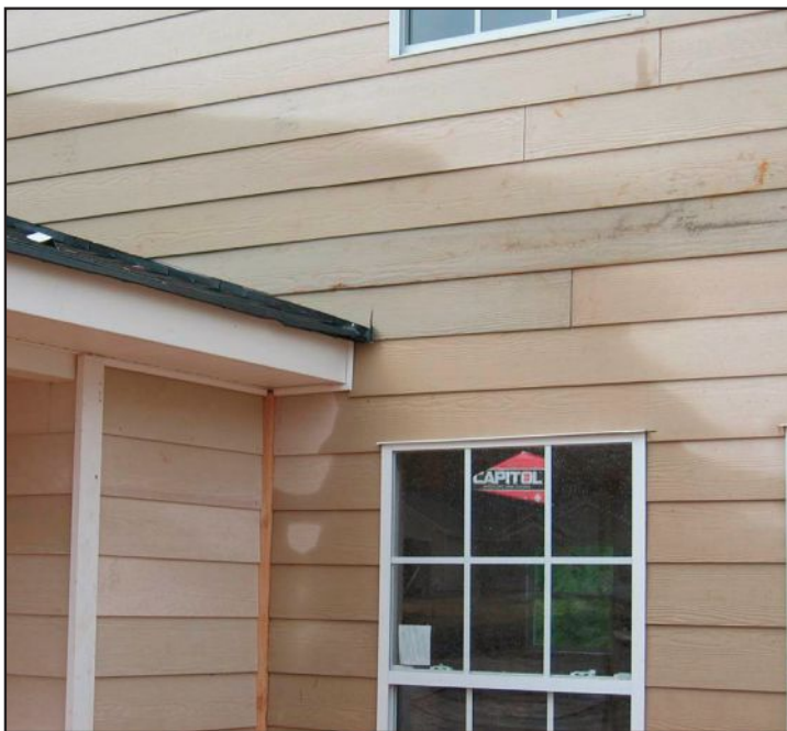
Without flashing, as in the image on the left, it is a challenge to control the rainwater because most multi-family buildings have transitions between materials or wall assemblies.
