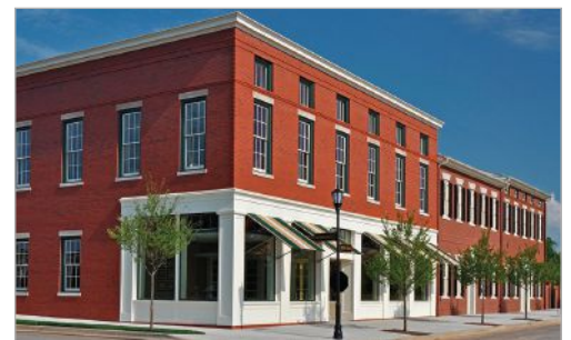
CMTA Headquarters, Louisville, Kentucky. Photo courtesy of Nudura and CMTA Consulting Engineers.
