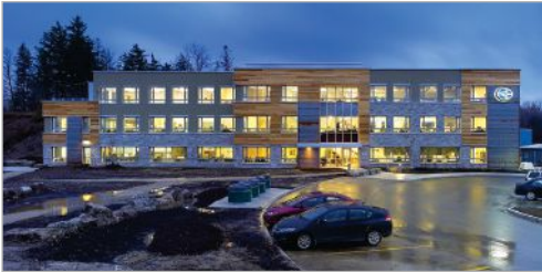
Enermodal Engineering Headquarters, Kitchener, Ontario. Photo courtesy of Nudura and Enermodal Engineering.
