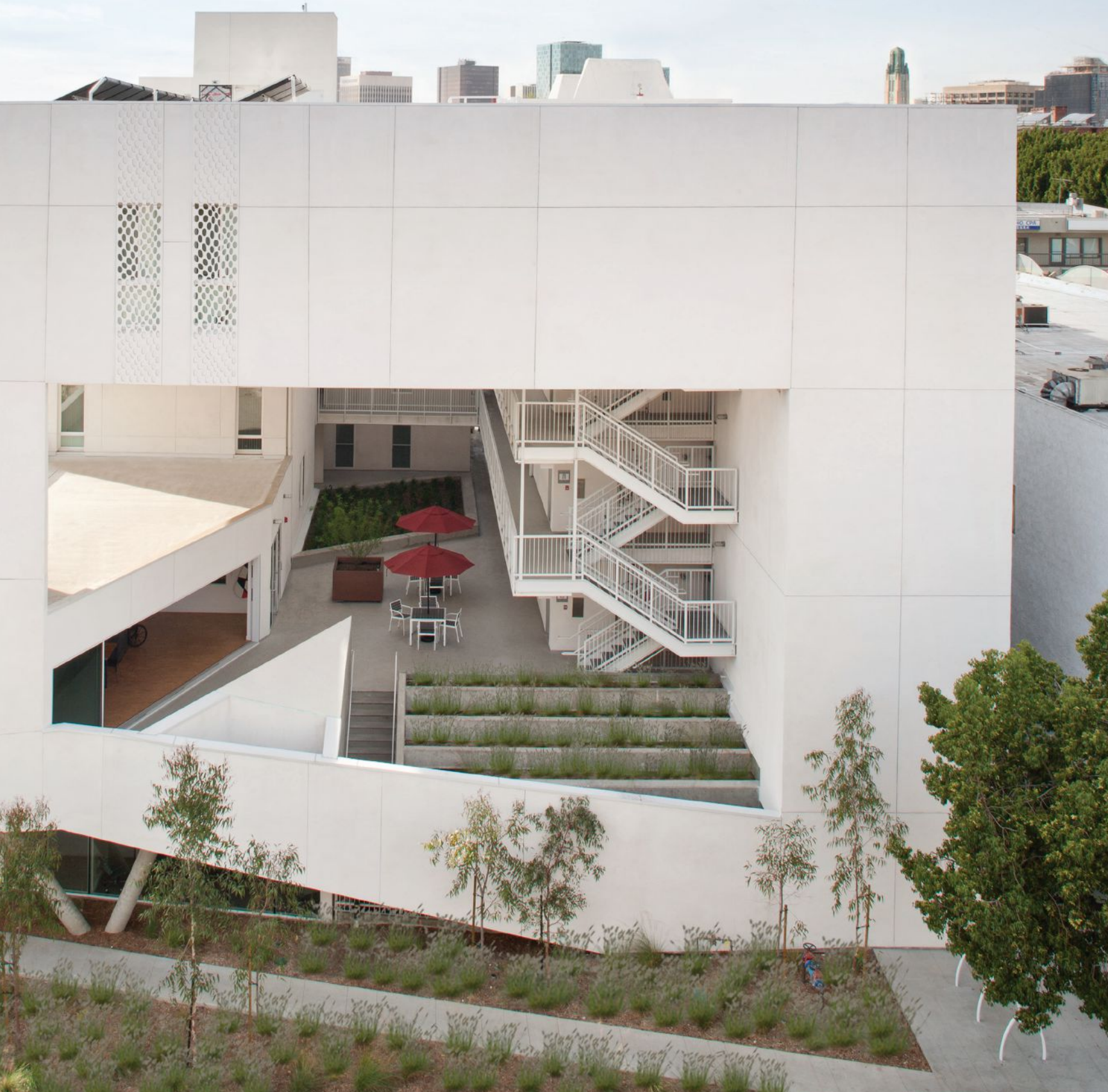
Exterior view from east, showing interior, second-floor courtyard
