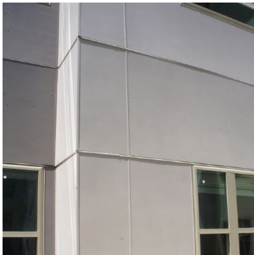
Extruded aluminum adds durability and longevity to construction that other trim materials such as polyvinyl chloride (PVC), and the galvanized steel shown in this image, lack.
