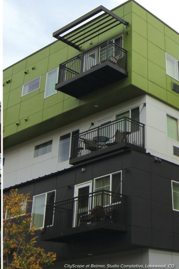
CityScape at Belmar, Studio Completiva, Lakewood, CO
