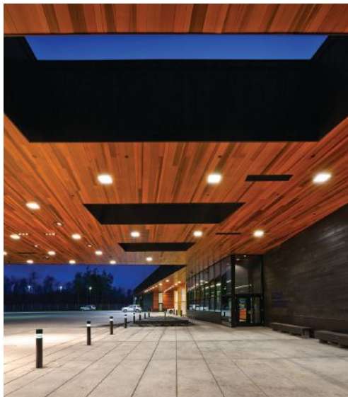
ABOVE: The port of entry overcame unique construction, environmental, and security challenges to produce a beautiful and sustainable project.
