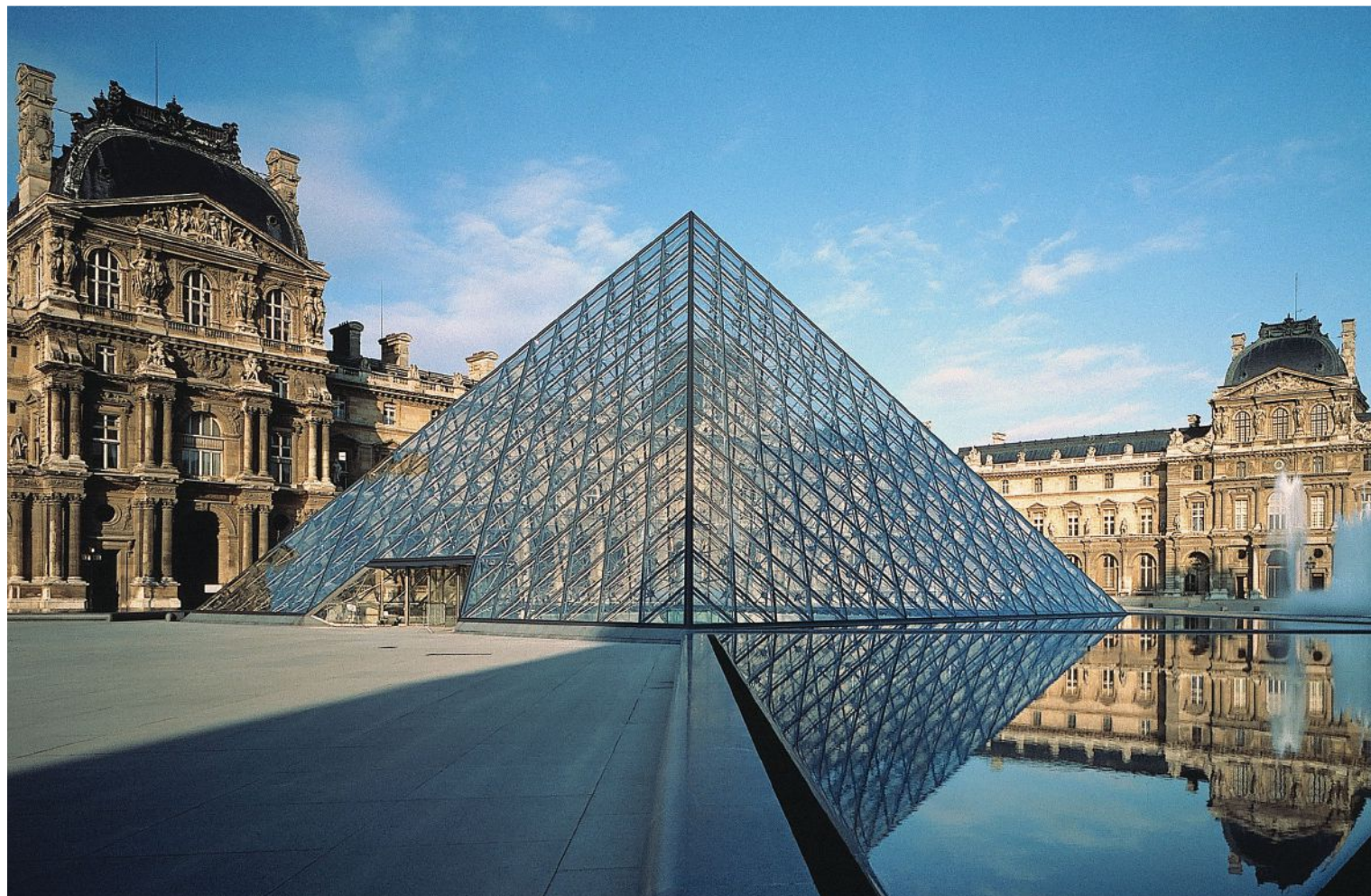
The Pyramide du Louvre was designed to divorce itself from the surrounding buildings while also employing low-iron glass to limit distorted views of the Louvre Palace.
