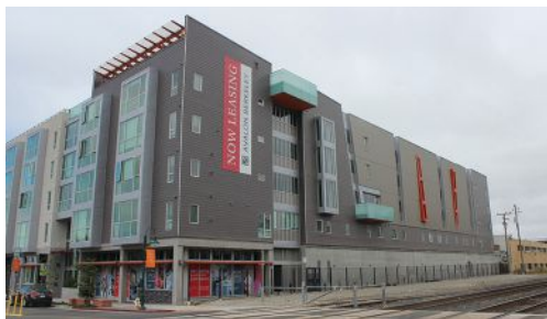
Using aluminum trim over panel joints on multifamily exteriors is an architectural element and is a way of expressing the joints and defining their deliberate placement. It adds a level of architectural refinement, particularly wherever fiber cement panels or lap siding is specified.
