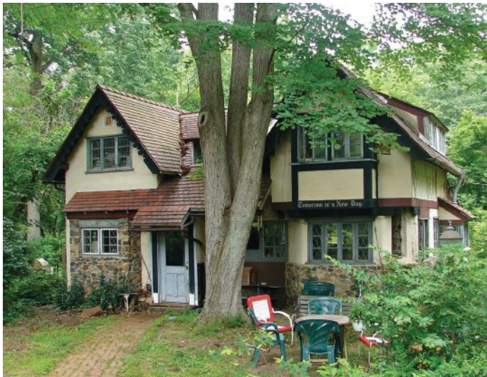
A house in Arden, Del.
