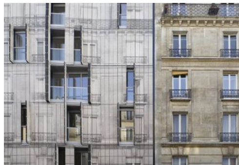
Residential 147 Chartier-Corbasson Architectes
