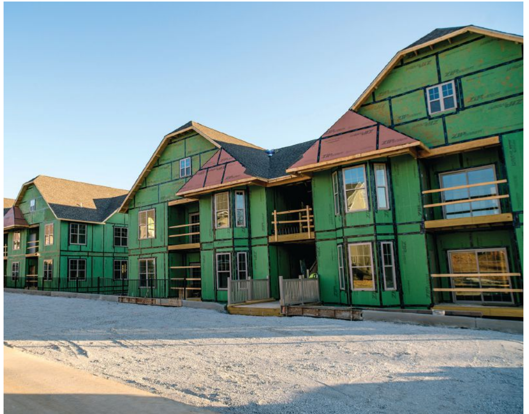
Bramblett Hills Apartments includes 218,000 square feet of ZIP System® panels.
