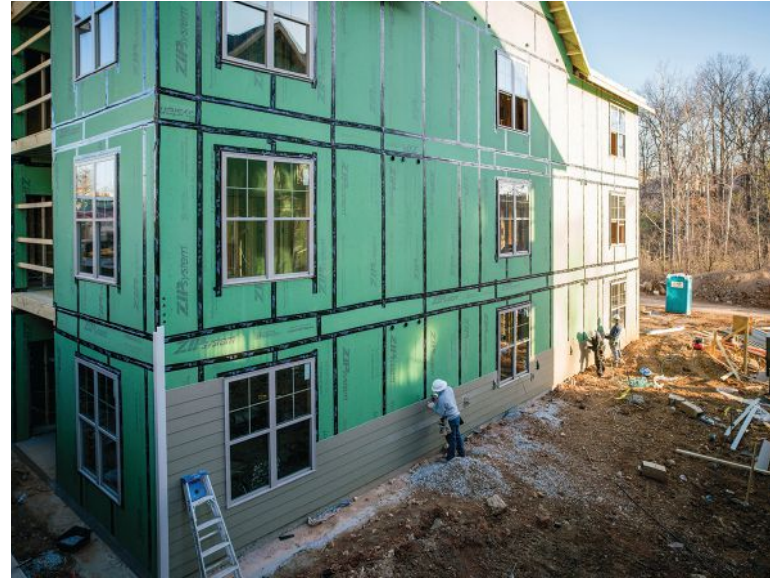
With a built-in water resistive barrier, ZIP System® sheathing and tape saves installation time by eliminating housewrap.
