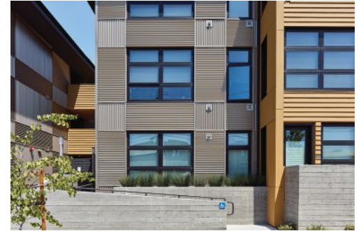
The various profiles and sizes of trim helped architects integrate the different materials into the façade. At 3900 Adeline, trim options allowed developers to cut down larger cement panels to create an intermediate scale, as well as to reorient the corrugated metal panels.
