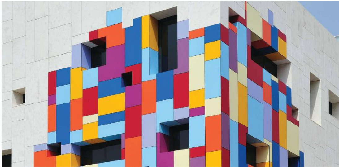
Centro Cultural CA DON JOSÉ Canals, Spain Rainscreen facade clad with Trespa® Meteor® Hector Luengo Arquitectos
