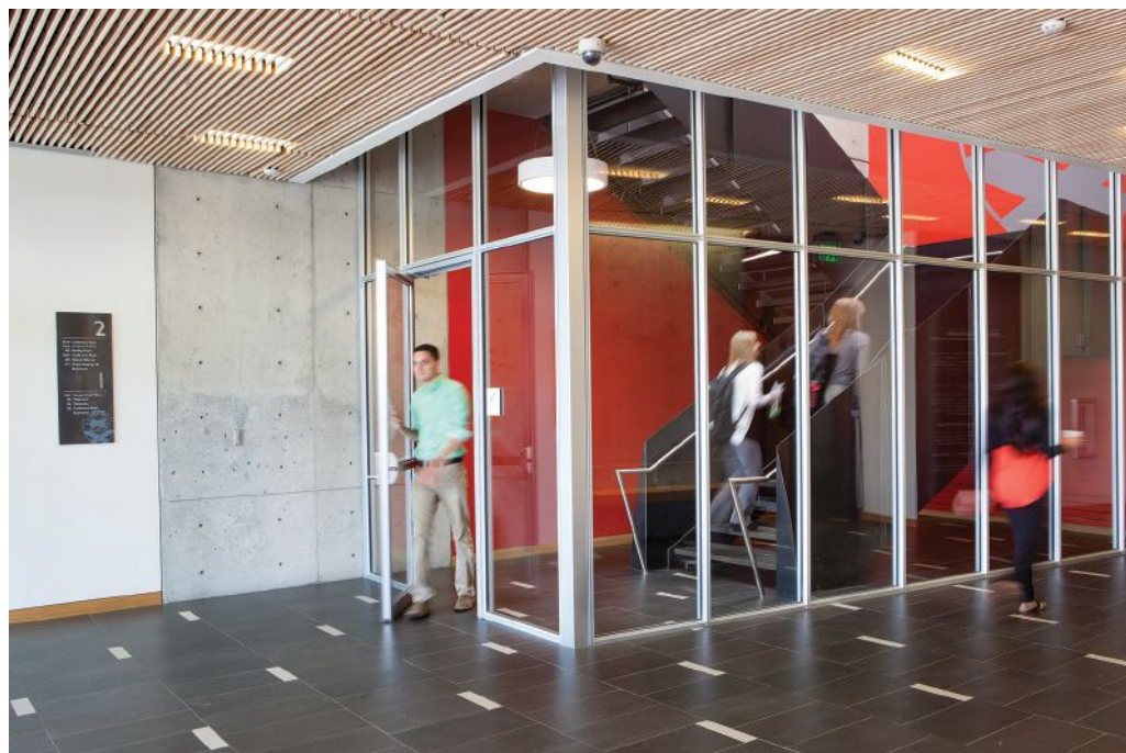
Fire-rated transparent wall panels can satisfy stringent building codes and exceed 25 percent of the total wall area, creating light-filled and open pathways in critical fire areas. Photo courtesy of Heidi Gumula—DBWW Architects
