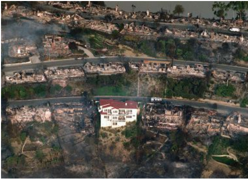
Noncombustible exterior finishes including stucco walls along with concrete roof tile helped protect this home during a 1993 wildfire in Laguna Beach, California (AP Photo/Douglas C. Pizac).
