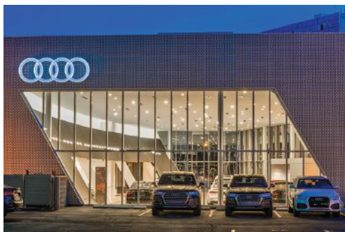
A fire-rated glazing system provides stylish lot-line protection, while its strength allows for 21-foot free spans.
