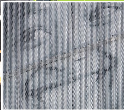
7/8-in. perforated corrugated panels overlay the graphic
