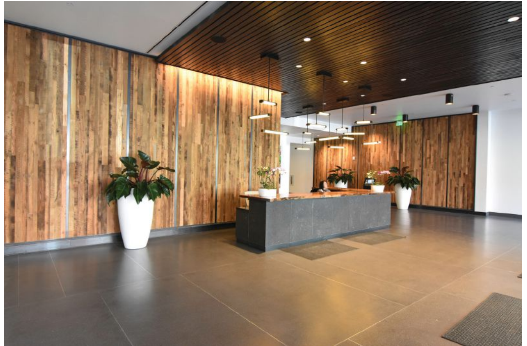
Figure 3. A subtle satin sheen on a grey dyed and polished concrete floor adds sophistication to a lobby reception area. Photo courtesy of Colorado Hardscapes, Denver, CO.
