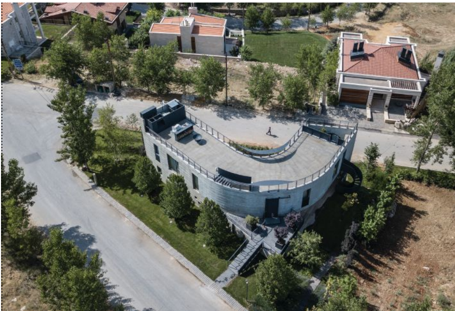
The boomerang-like form of the house's upper level is designed to maximize views.
