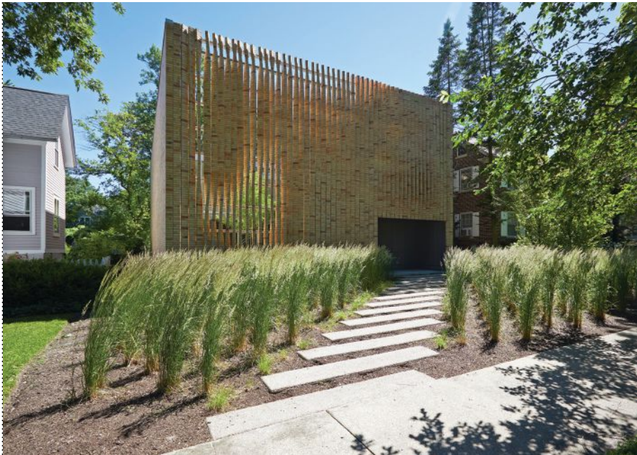
Street façade with brick screen
