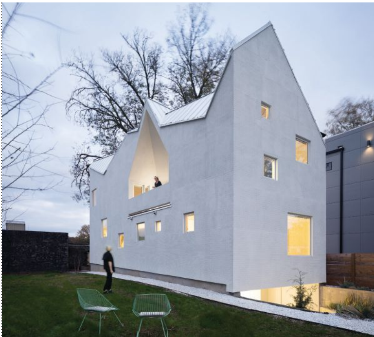
View from northwest, showing cementitious stucco finish with embedded glass beads.
