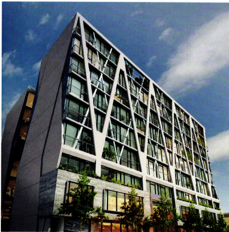
Figure 1: Rowan, San Francisco. One of San Francisco's newest and sleekest residential structures uses a giant, zigzagging concrete exoskeleton and stands out from other buildings. The exterior is for much more than show—it negates the need for interior columns, maximizing the interior space for residents. Concrete on the project used high volumes of fly ash to reduce environmental footprint.
