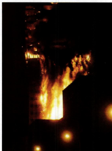
This photo shows the results of "leapfrog" fire propagation.
