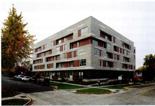
COOL FOR SCHOOL | University House Arena District, Eugene, OR Podium construction can be an efficient and cost-effective way to meet the rapidly growing demand for student housing across the country. This 109,600 square-foot student housing project includes five stories of wood-frame construction over a concrete podium achieving an attractive yet affordable design. PHOTO CREDIT: Lincoln Barbour | ARCHITECT: Mahlum Architects
