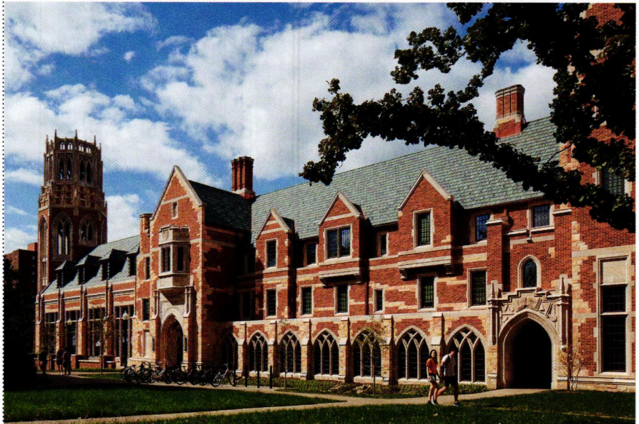
South façade, showing brick detailing, slate-mimicking ceramic roof tiles, and chimneys that conceal plumbing and mechanical systems.
