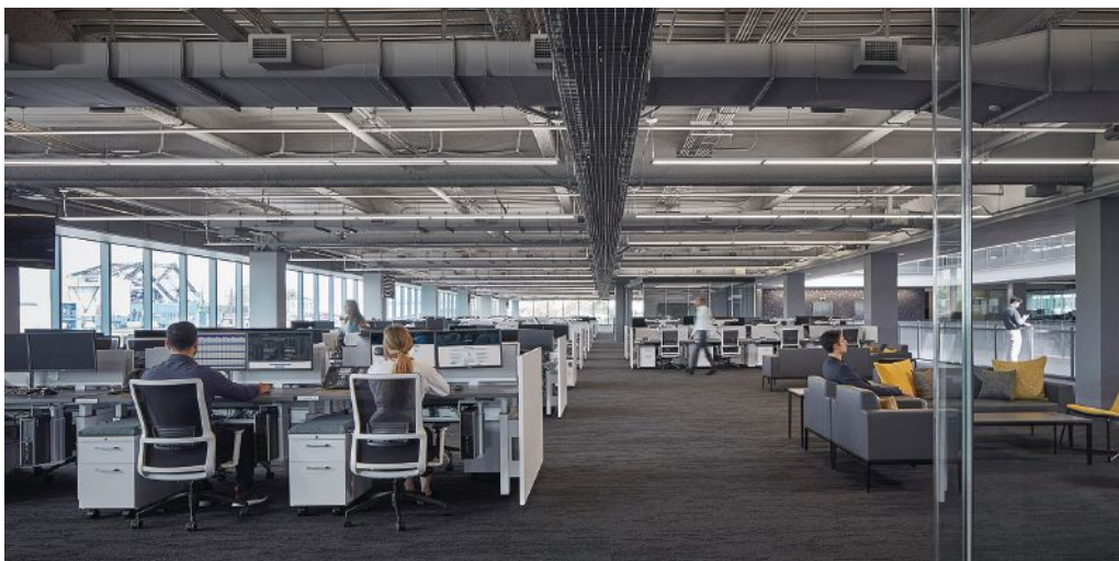
Steel framing maximizes open office design by providing long spans between columns as exhibited by the C.H. Robinson Midwest Headquarters in Chicago, IL.
