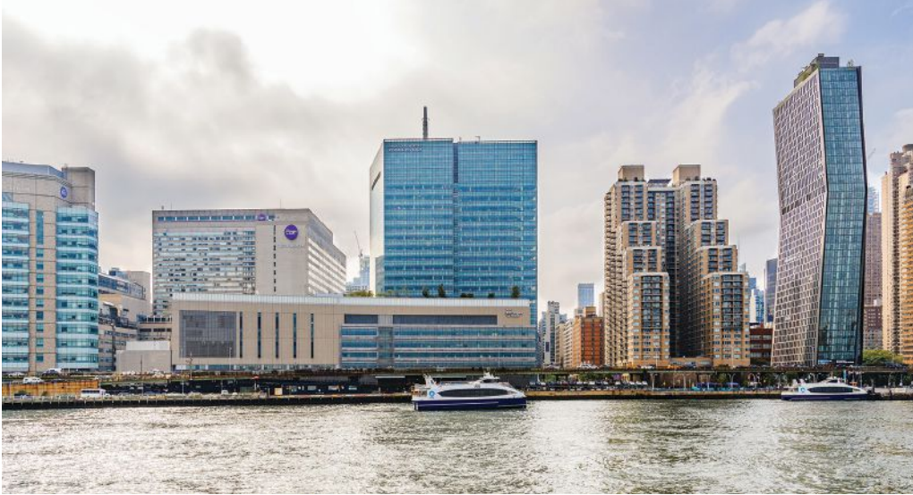
NYU Langone Health Helen L. and Martin S. Kimmel Pavilion is located in a dense urban environment with sound emanating from the street level, an adjacent freeway, nearby river traffic, and underground commuter train tunnels in New York, NY. Photo Courtesy of LERA Consulting Structural Engineers/Fadi Asmar
