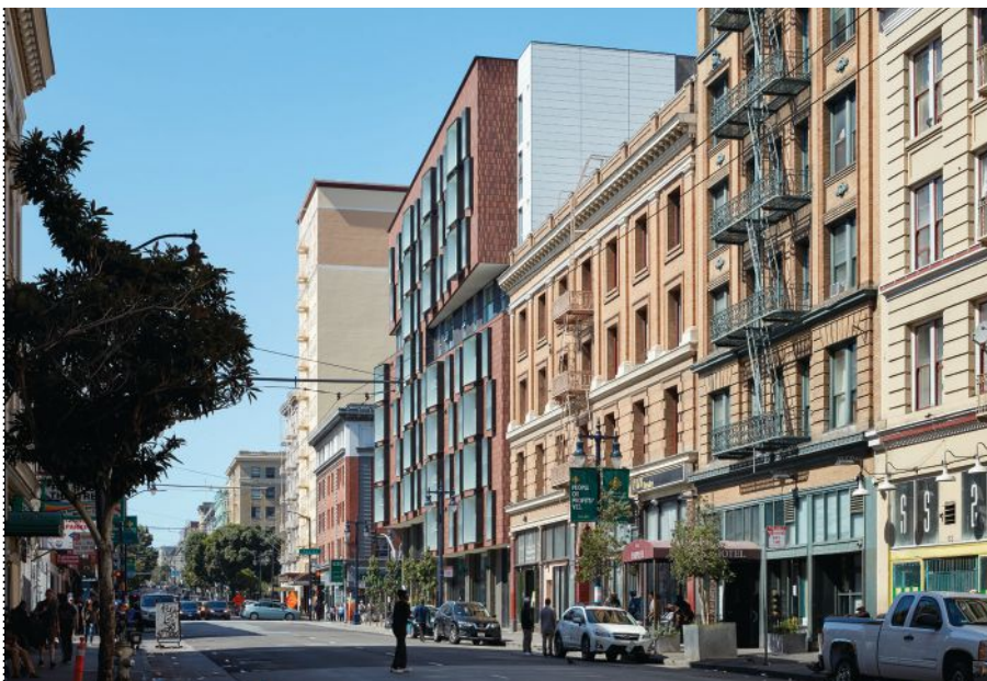
The aluminum window surrounds of 222 Taylor provide shading to help minimize energy consumption.
