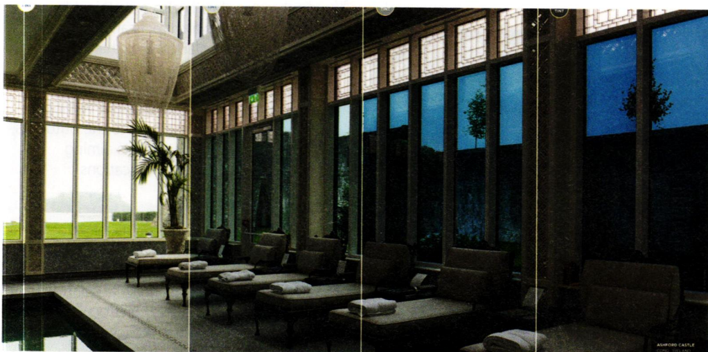
The different tint states of electrochromic glass in action at Ashford Castle in Cong, Ireland ©Sean Conboy.
