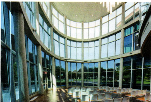
Electrochromic Glass tints to control heat and glare, making the space usable again.
