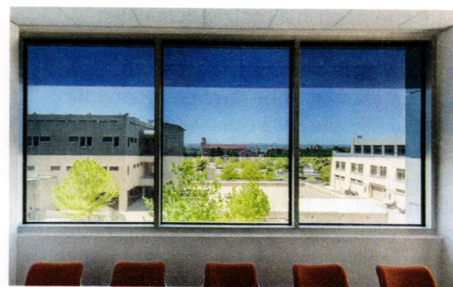
In-pane zoning on display at the University of New Mexico Farris Engineering Center.
