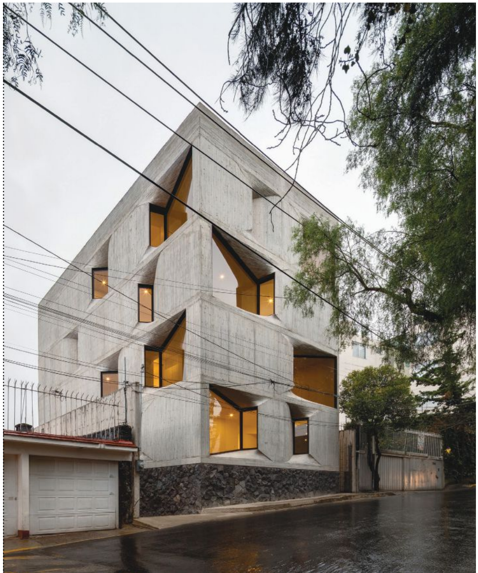
Twenty-two windows based off of five different molds punctuate DL1310's cast-concrete façade.
