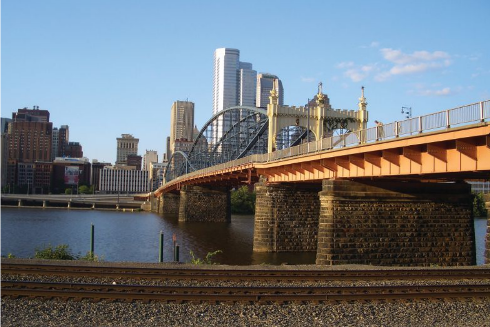
One of the traditional uses for a 2K polyurethane coating is a weather, chemical, and color stable topcoat in a multi-coat system for bridge steel corrosion protection.
