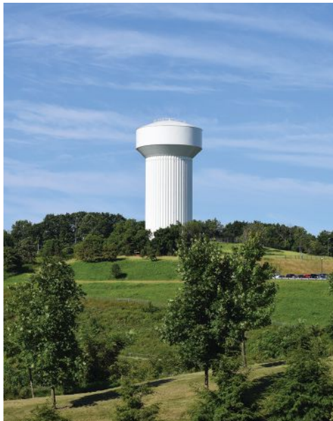
This municipal water tower was coated 26 years ago with an all-polyurethane coating system and has maintained excellent corrosion, color, and gloss properties.
