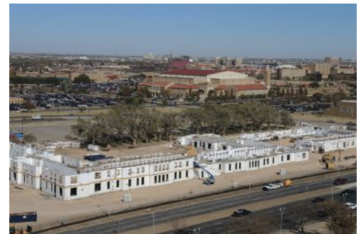
West Village Student Housing Under Construction. Image courtesy of Fox Blocks
