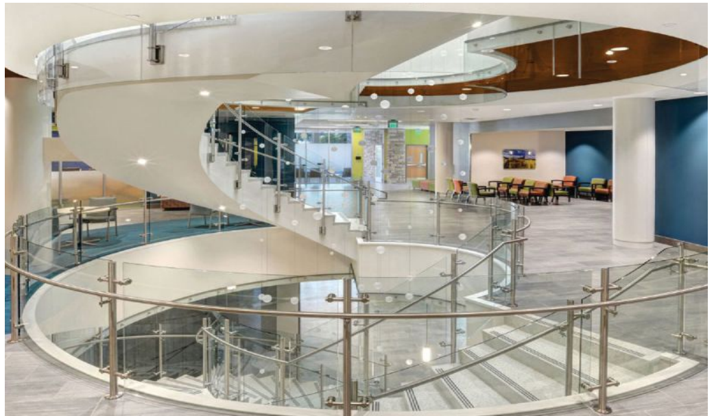
Using 3-D laser scanning, Trex Commercial Products precisely engineered the custom stainless and glass railing system for this stunning spiral staircase at Colorado State University Health and Medical Center. Photo credit: Trex Commercial Products
