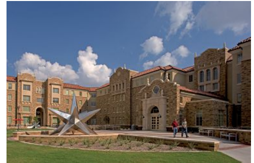
West Village Student Housing. Photo courtesy of Mackey Mitchell Architects
