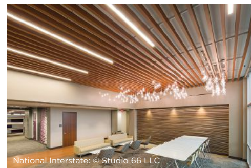
Metal ceiling systems can be clad in both real wood veneer or decorative wood-look options.
