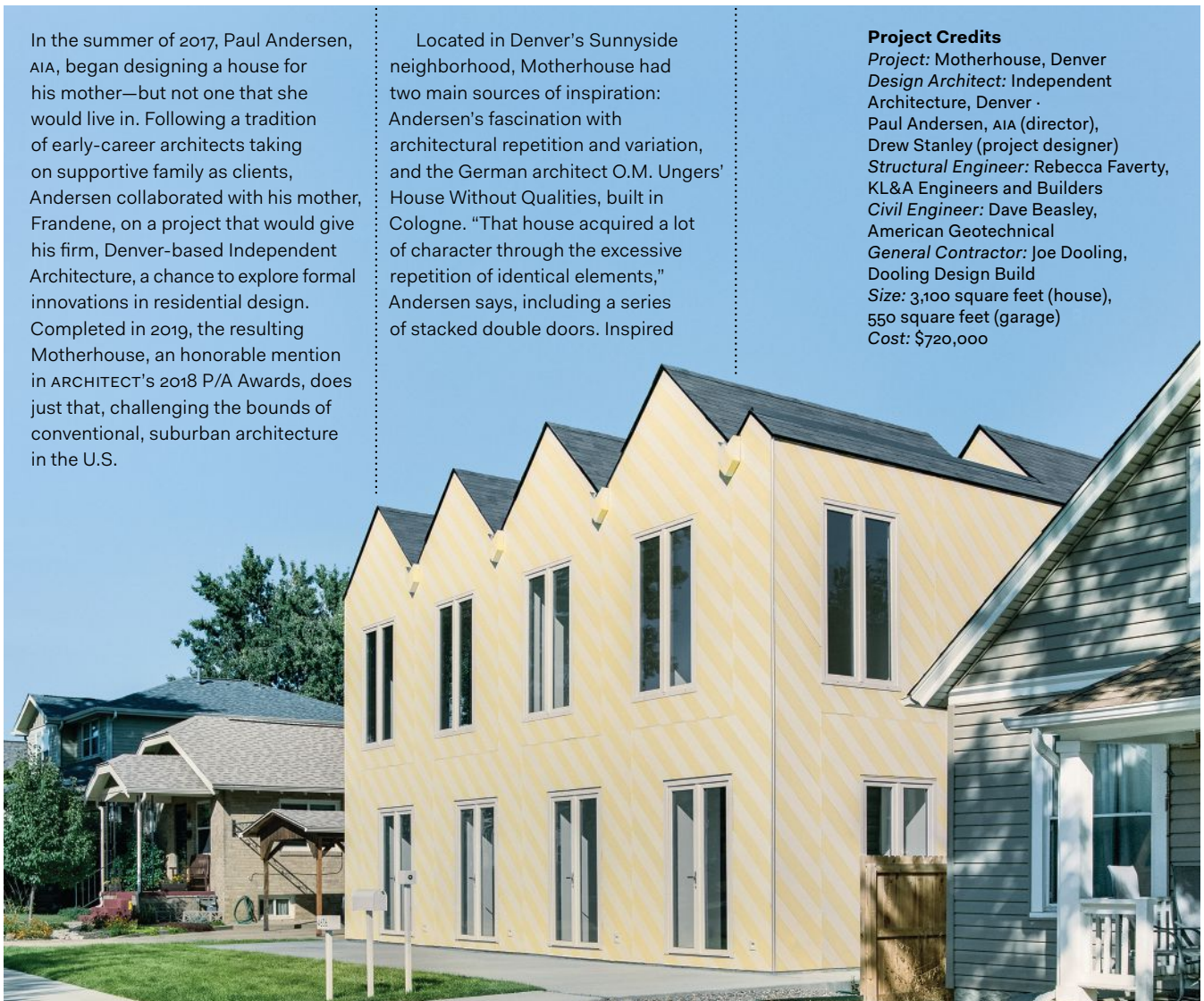
Motherhouse's candy-striped envelope comprises yellow-and-white-painted Boral TruExterior nickel-gap siding made from polymers and fly ash.
