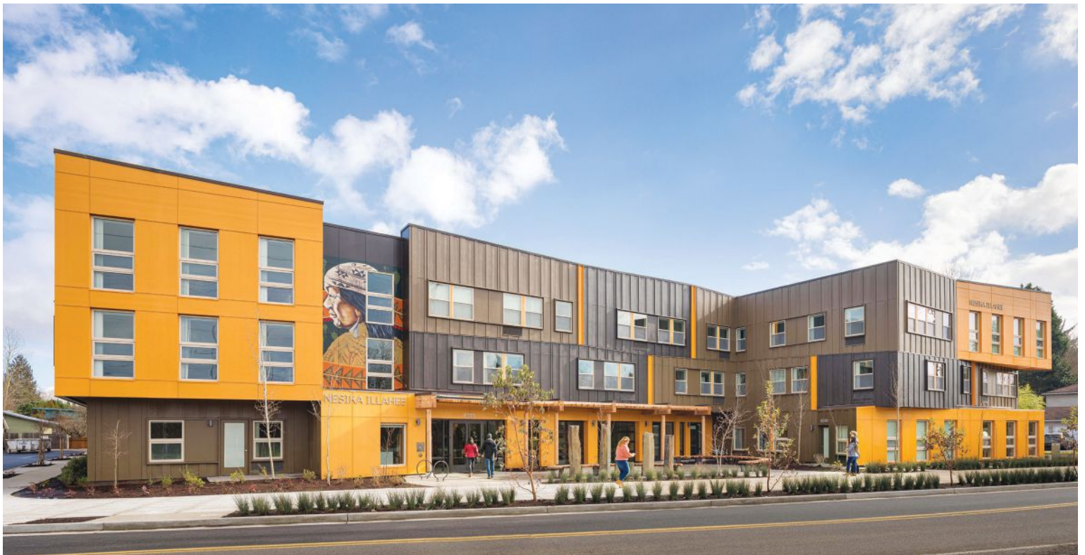
Nesika Illahee, a Native-focused affordable housing development in northeast Portland, Ore., was brought to fruition by Community Development Partners
