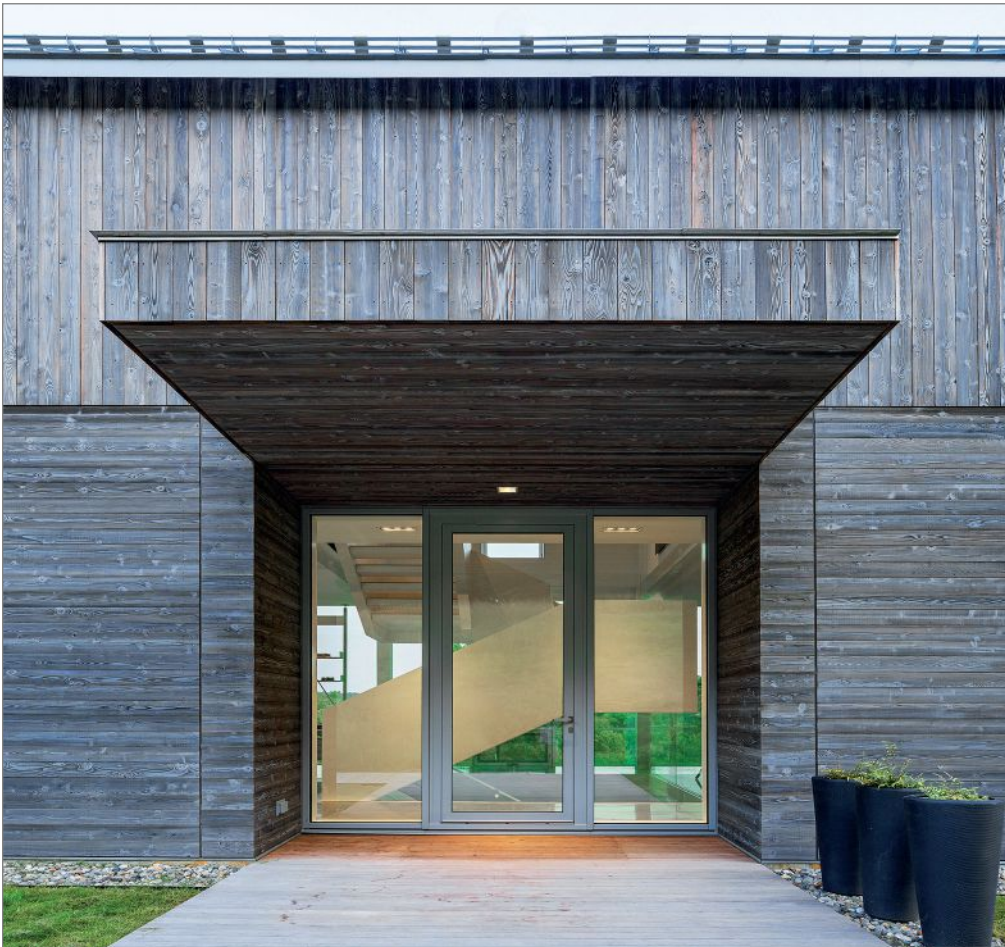
Western red cedar siding provides a wealth of options to provide the perfect look for a home, as it can be finished to complement all styles of buildings from modern to traditional to rustic. Bank Barn. Architect: Birdseye. Photography: Jim Westphalen Photography, Birdseye.
