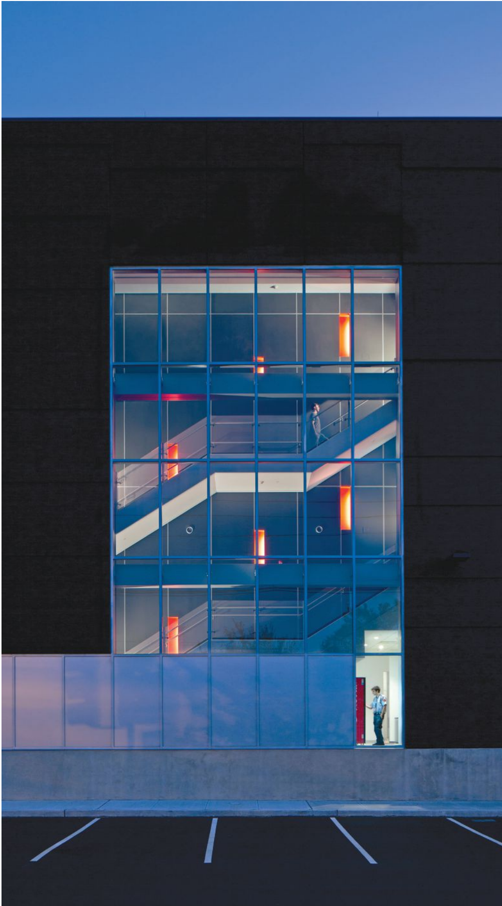
The NY5 data center in Secaucus, New York, was designed by Sheehan Nagle Hartray Architects.
