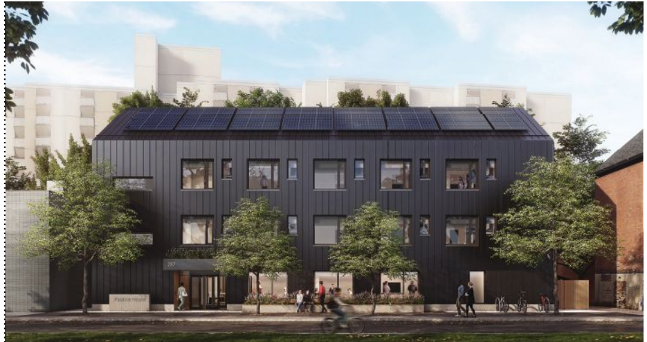
As part of its Passive House Certification goals, the new Hamilton residence will feature photovoltaic panels on its south-facing roof.
