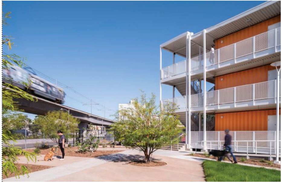
Constructed in just six months, the Hilda L. Solis Care First Village in Los Angeles features three kinds of modular elements: shipping crates, conventional prefabricated units, and single-story trailers.
