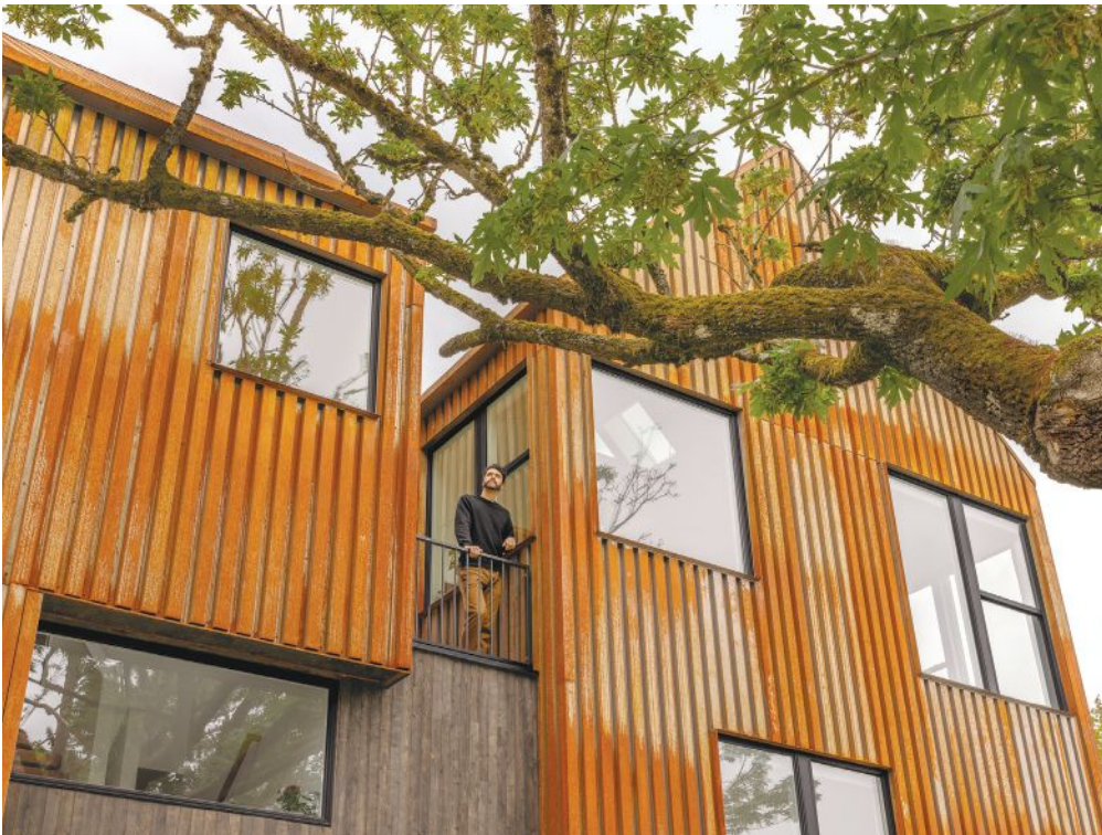
The context of the existing neighborhood was an important consideration in Hybrid’s design.
