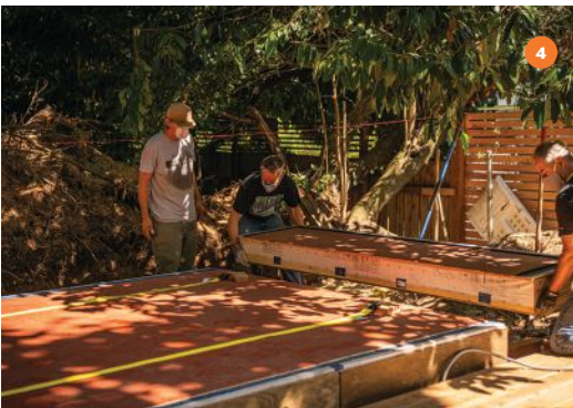
1. Block Home 0010, built in 2020 in Seattle’s Central District neighborhood, was the Block Project’s first completed structure following 2019 redesign efforts. 2. Volunteers transform Havelock wool into insulation at the Block Project workshop. 3–4. Thanks to prefabricated elements, Block houses can easily be constructed on-site by small teams of four people. 5. A drawing for the redesigned Block Home. 6. A Block Project construction team at work.
