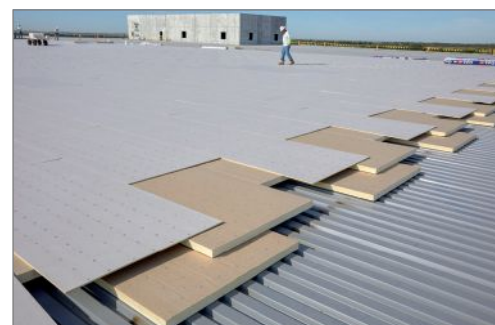
Staggered and offset insulation board joints.
