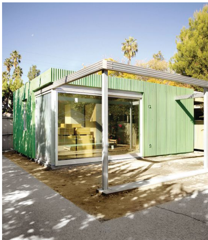
The Ranchito Toy Box, designed by architect Linda Taalman—founder of IT House and Taalman Architecture—is an IT Box, a 360-square-foot ADU that converts an existing carport to a Junior Accessory Dwelling Unit. It is one of six IT House Standard Plan options preapproved for the city of Los Angeles.
