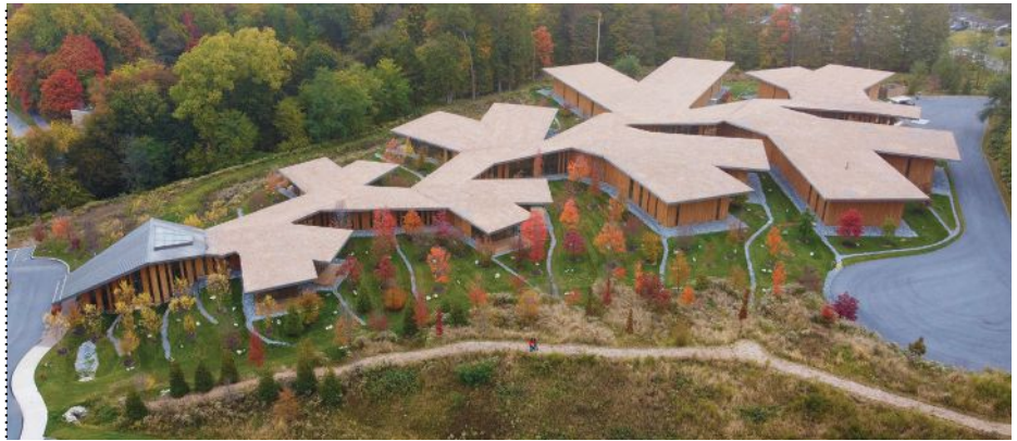
Located in Harrisburg, Pa., the JST Harrisburg Production Center takes the form of a branching root system and features exterior cypress wood siding.
