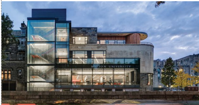
For Boston University's Alan and Sherry Leventhal Center, the local firm Goody Clancy completed an adaptive reuse of a 1953 International-style building.
