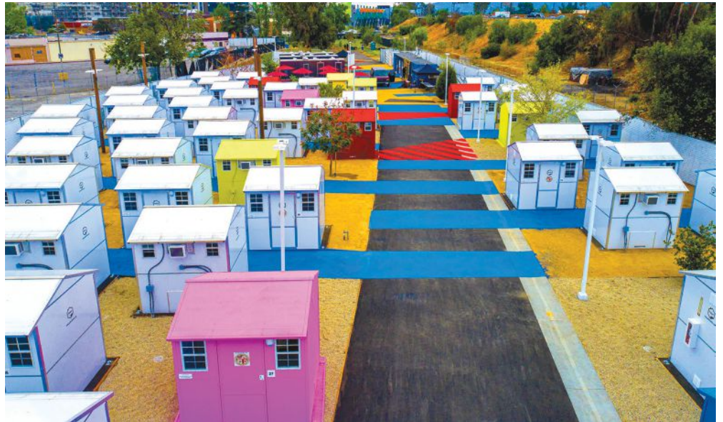
Project architect Michael Lehrer, FAIA, says that one of the benefits of the Tiny Homes Villages is the speed with which they can be constructed.
