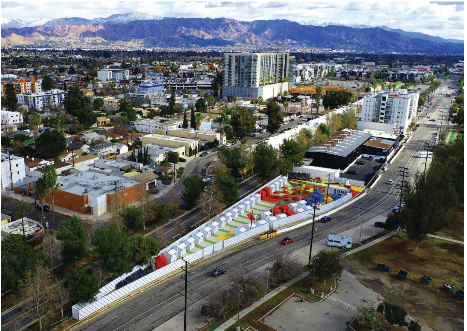
Chandler Boulevard Bridge Home Village, completed in February 2021, was the first Tiny Homes Village project.
