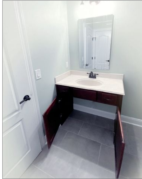
While they look like traditional cabinets on the outside, these open fully and have no exposed piping underneath so that wheelchair users can easily access the sink; this is a perfect example of the Size and Space for Approach and Use principle. Photo courtesy of Paragon Building Group.
