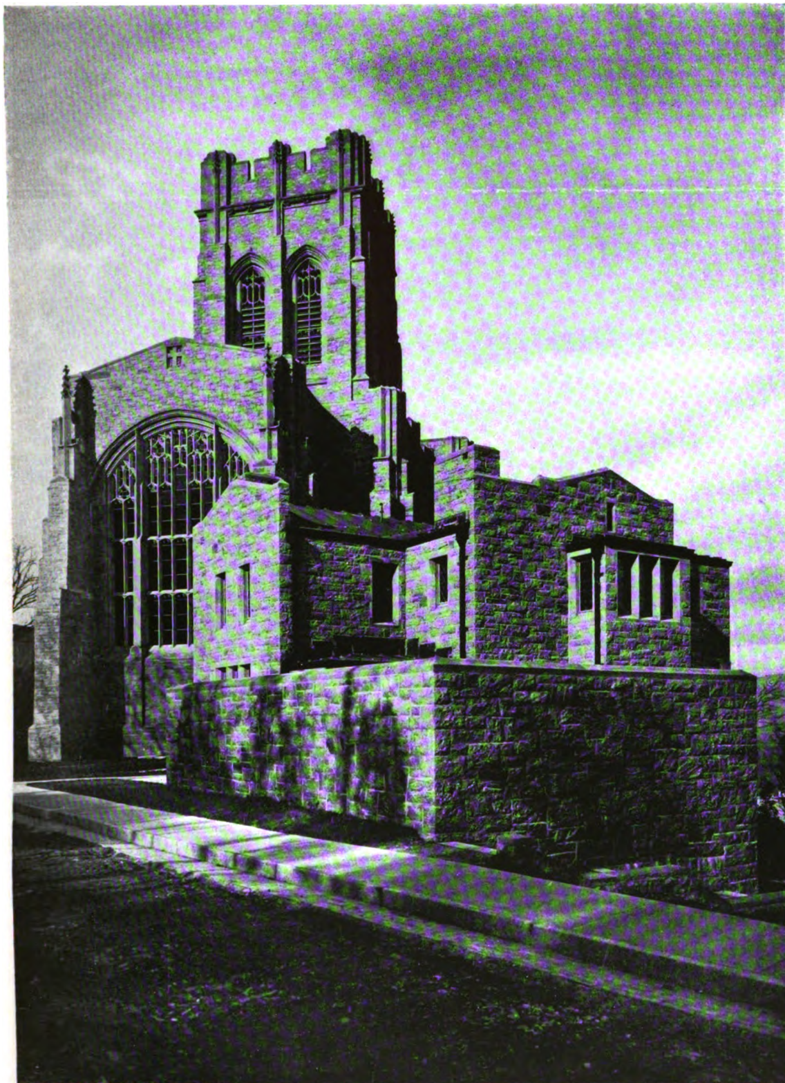
THE CHAPEL AND THE CHAPLAIN'S QUARTERS FROM THE SOUTH
