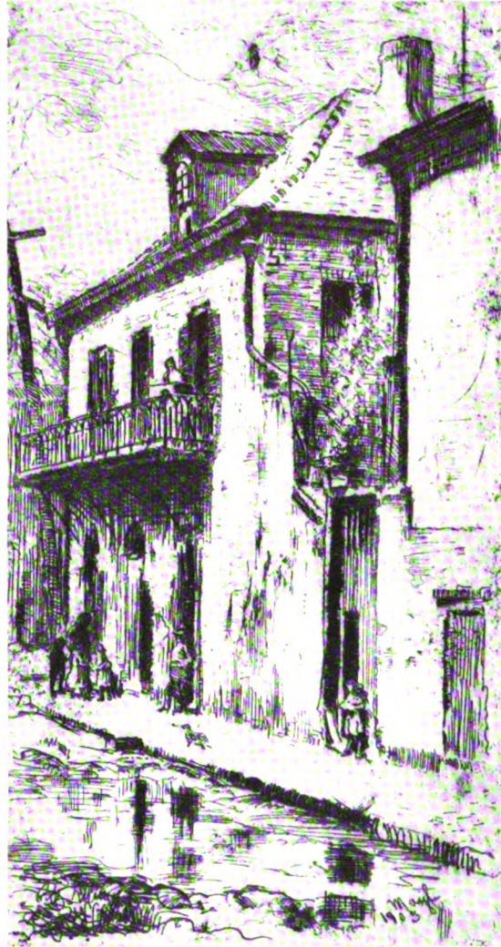
OLD HOUSE SHOWING THE EFFECT OF STUCCO After an etching by R. B. Mayfield
