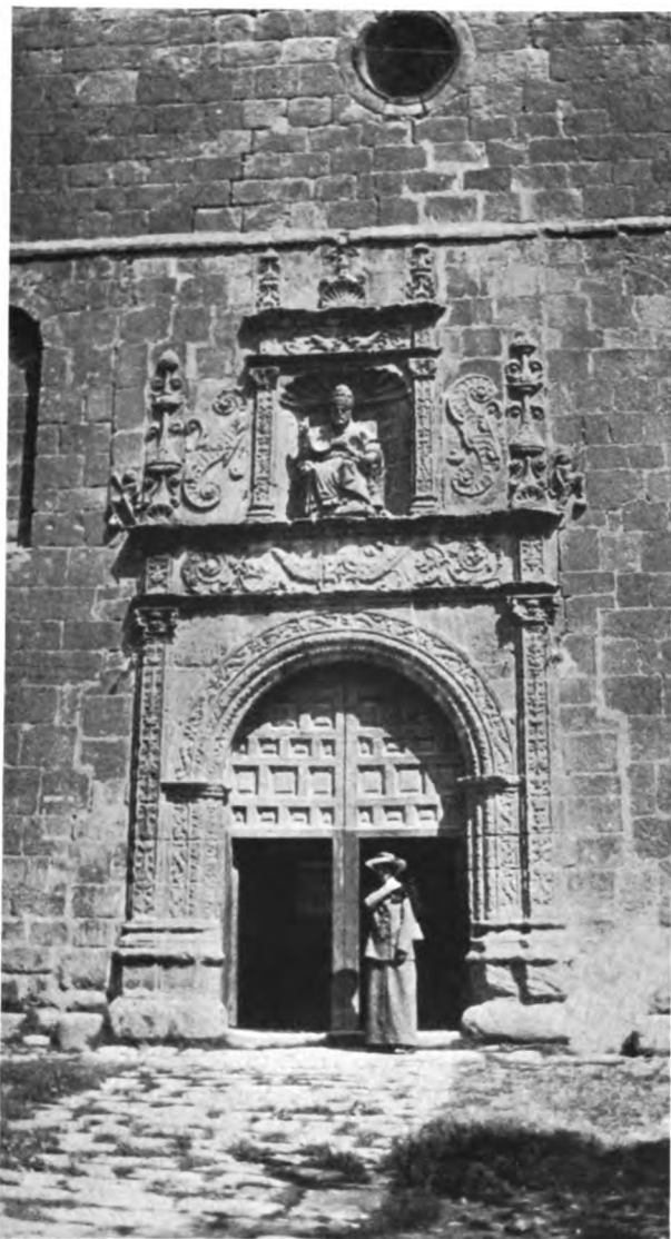
DOORWAY, S PEDRO
