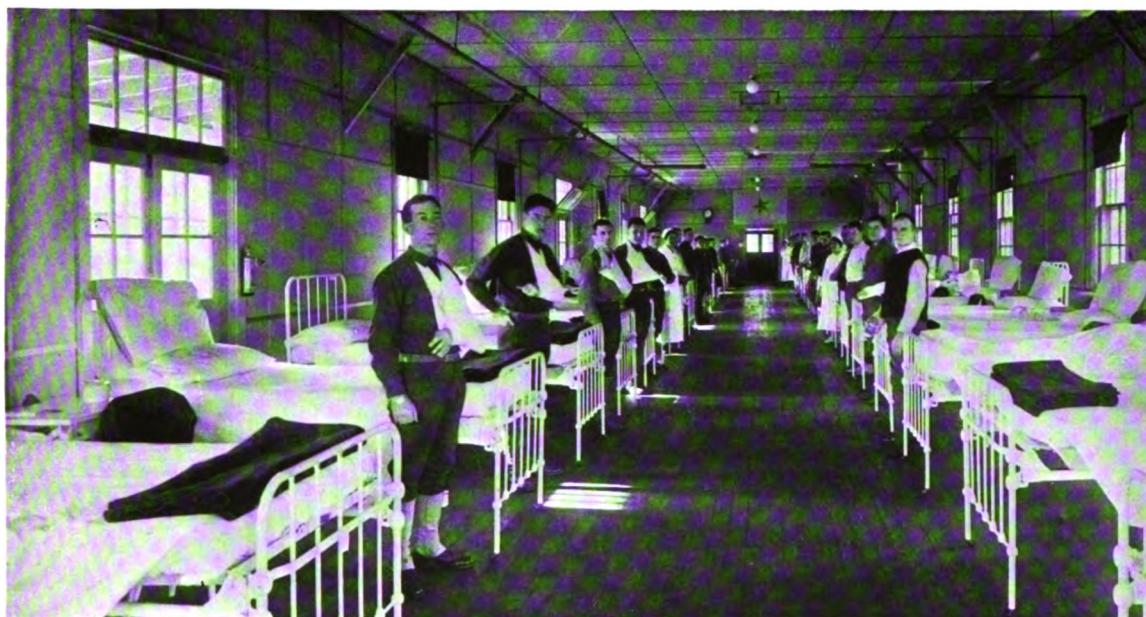
INTERIOR OF GENERAL WARD PAVILION K-1
