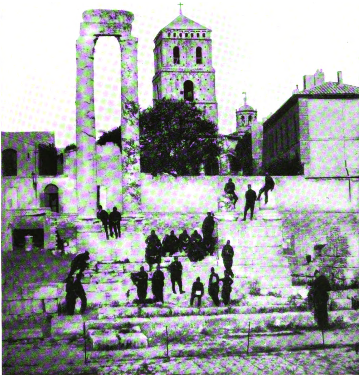
A. E. F. SCHOOL OF ARCHITECTURE.—FIELD WORK CLASS AT THE ROMAN THEATER, ARLES
