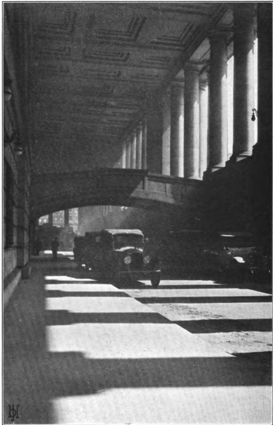
PENNSYLVANIA STATION, NEW YORK CITY—31ST STREET CAB DRIVEWAY After a photograph by Ben J. Lubschez
