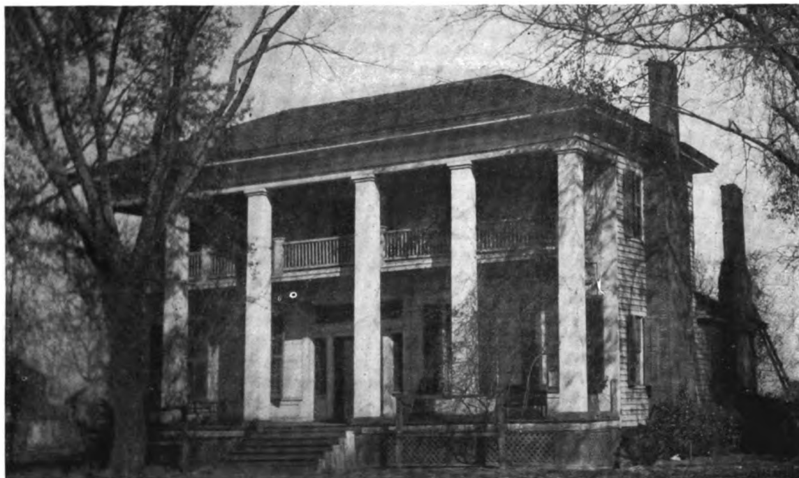
FIG. 5—A DOWNTOWN HOUSE IN TUSKEGEE, ALABAMA
