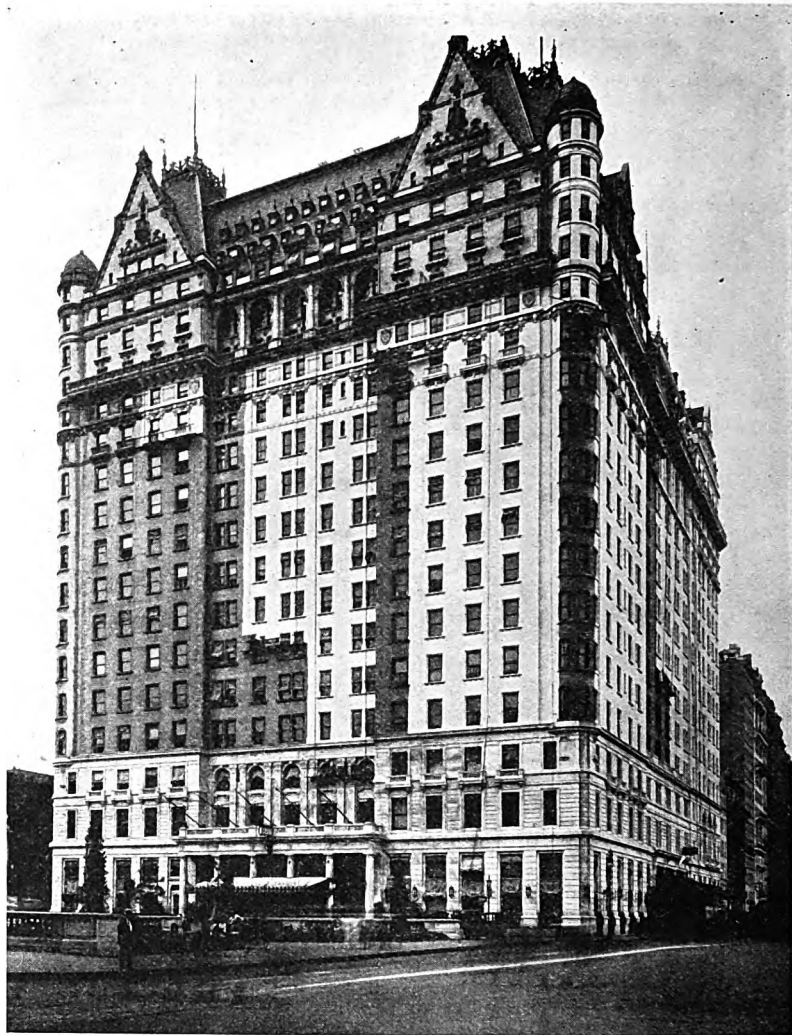
The Plaza Hotel during cleaning; Terra Cotta, glazed brick and marble
