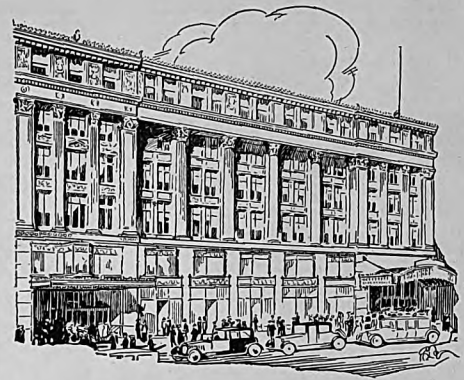
Capitol Theatre, Detroit, Mich. C. Howard Crane, Architect, Detroit Longacre Construction Co., Contractors Carey Asphalt Specification Roof
