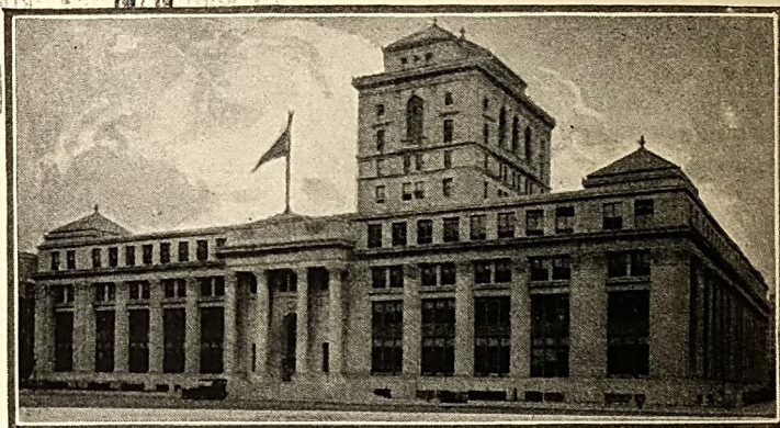
John Hancock Insurance Co. Building, Boston, Mass.—equipped with G-E Tumbler Switches. Parker, Thomas and Rice, architects. French and Hubbard, consulting engineers.
