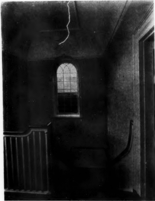
STAIRWAY IN THE HAMMOND-HARWOOD HOUSE—1770-1774. ANNAPOLIS, MD.
