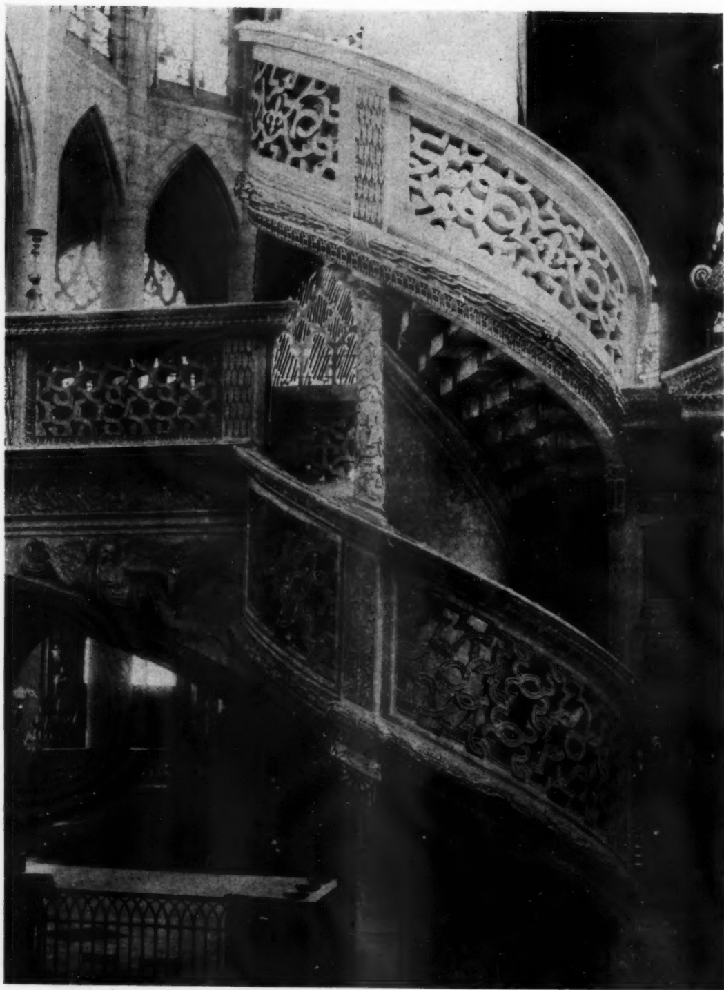
THE AMAZING AND FASCINATING, FLYING SPIRAL STAIRS WHICH LEAD, RIGHT AND LEFT, TO THE ROOD OF ST. ETIENNE DU MONT
