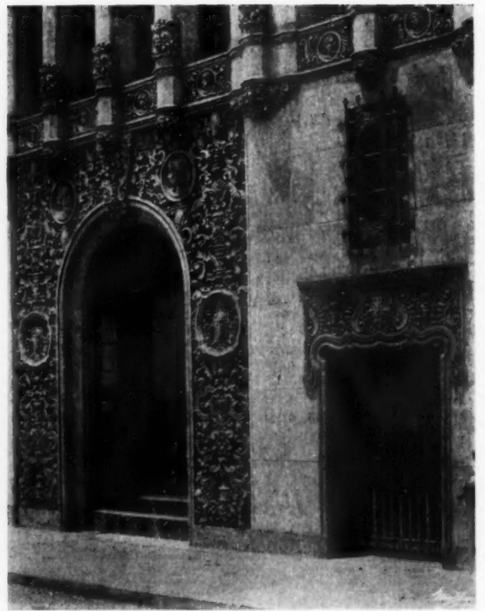
HOLLYWOOD TERMINAL WAREHOUSE MORGAN, WALLS & CLEMENTS, ARCHITECTS
