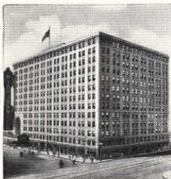
The Michigan building in Detroit which appreciates the advantages of Otis Elevator Modernization.
