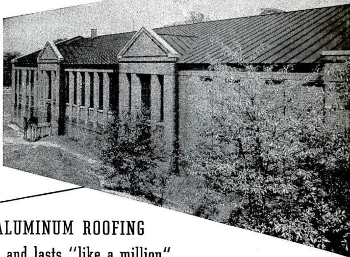
Aluminum roof on Shadyside Academy Junior School, Pittsburgh, Pa. Building designed by Rust Engineering Company of Pittsburgh.
