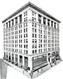
Slater Building, Worcester, Mass.
