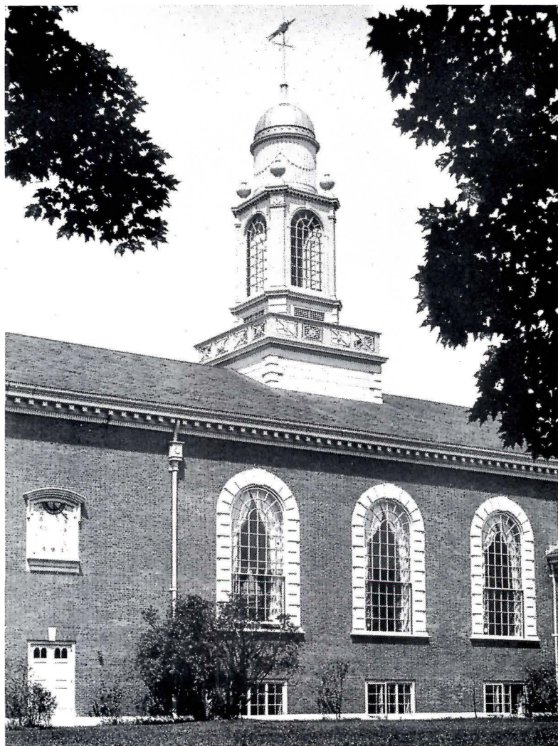
DETAIL OF BRYAN MEMORIAL TOWN HALL, WASHINGTON, CONN. CAMERON CLARK, F.A.I.A., ARCHITECT
