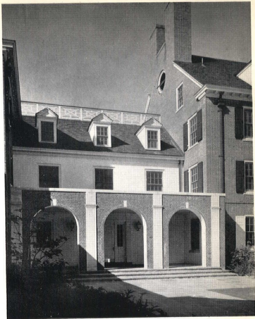
ENTRANCE PORCH, MEN'S DORMITORY MIAMI UNIVERSITY, OXFORD, OHIO CHARLES F. CELLARIUS, ARCHITECT
