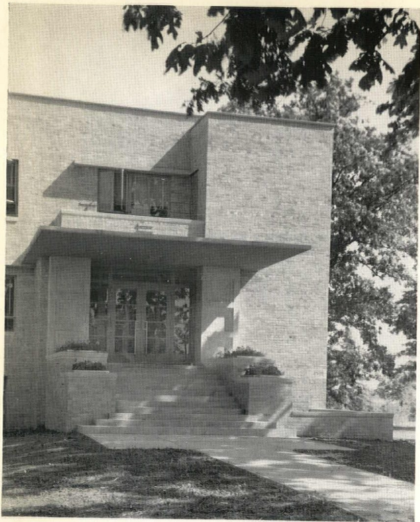
MAIN ENTRANCE, MAGRUDER MEMORIAL HOSPITAL PORT CLINTON, OHIO
