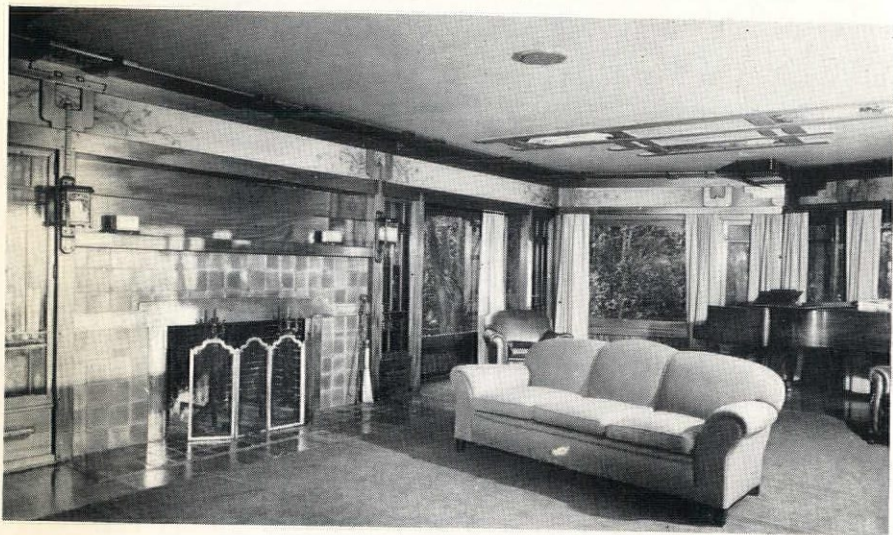
Flush ceiling-lights and integral curtain valances in the WILLIAM R. THORSEN HOUSE, Berkeley, 1908, are typical Greene & Greene details
