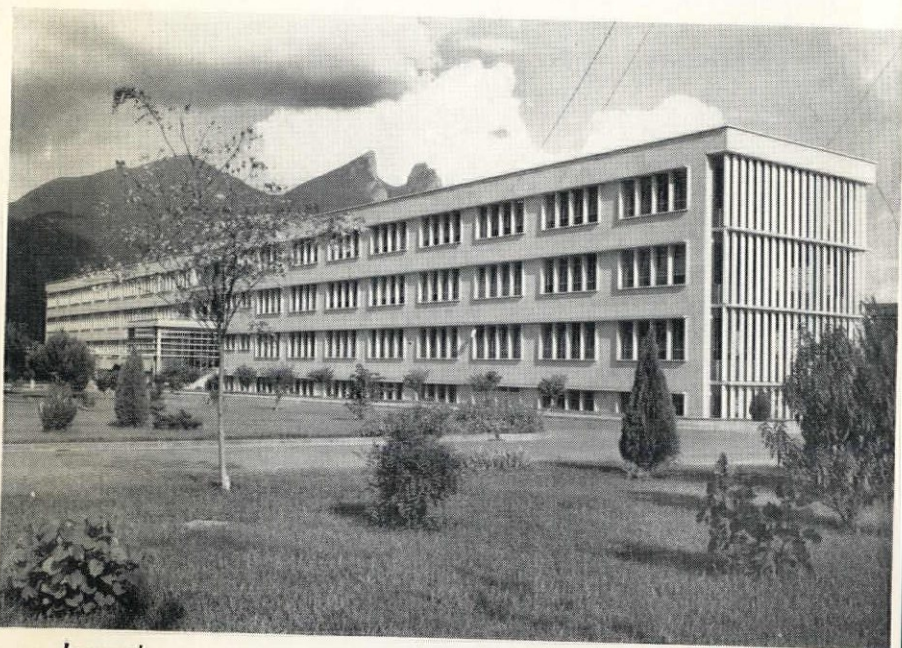
CLASSROOM BUILDING OF THE INSTITUTO La Silla Mountain in the background
