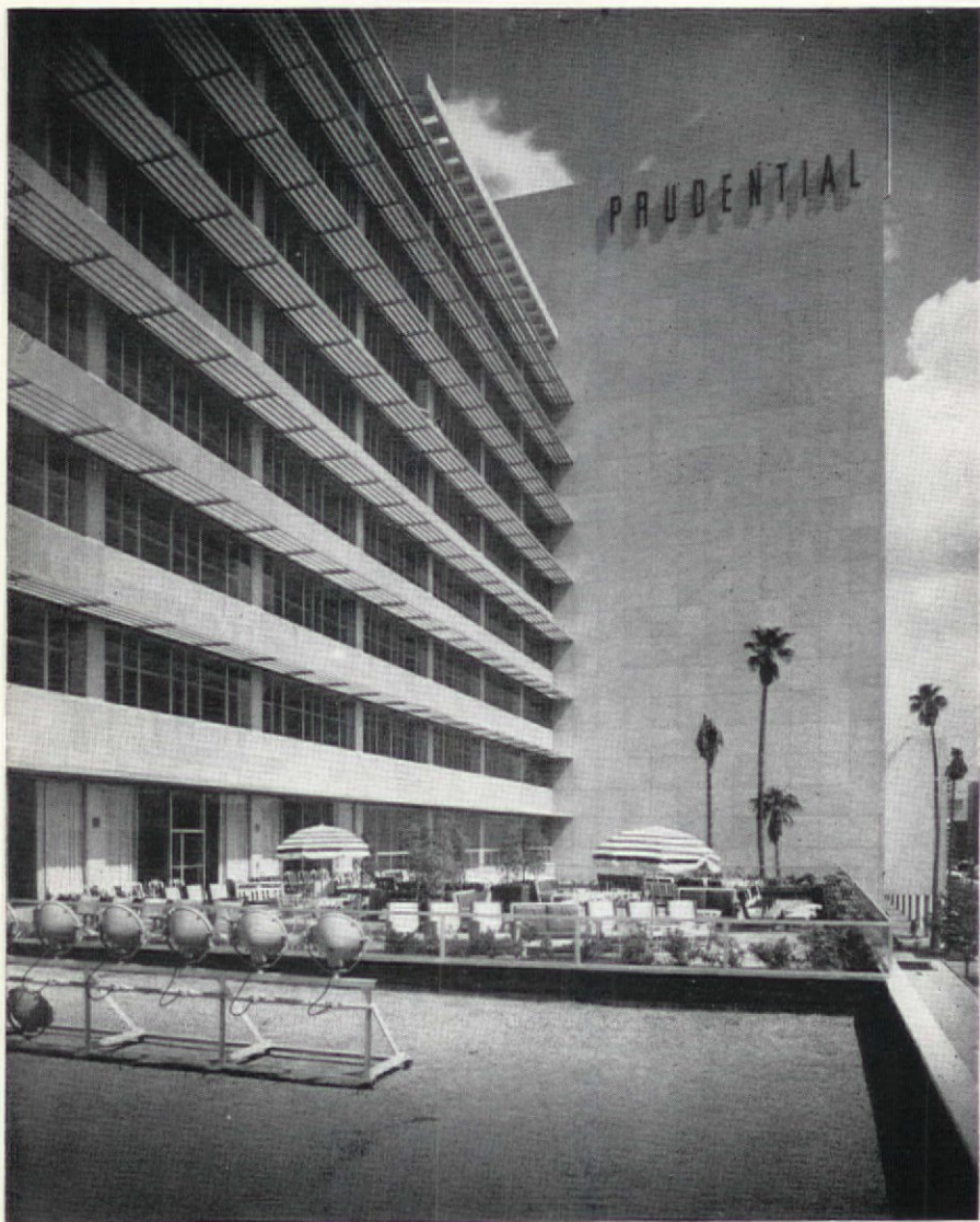
DETAIL OF PRUDENTIAL BUILDING, LOS ANGELES, CALIF. WELTON BECKET & ASSOCIATES, ARCHITECTS AND ENGINEERS
