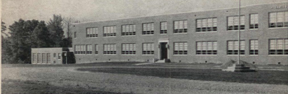
James Solomon Russell School, Brunswick County, Va. Total square footage — 67,356. Cost $524,870. Heating Contractors: W. J. Bloomfield & Son, Inc., Farmville, Va.
