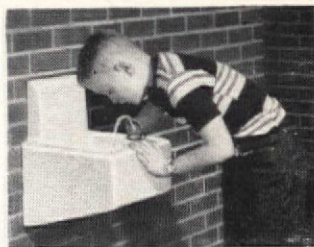
Crane school fountains are of highest quality vitreous china. This Crane Waterfall includes Crane's Purflo angle stream bubbler to prevent contamination.
