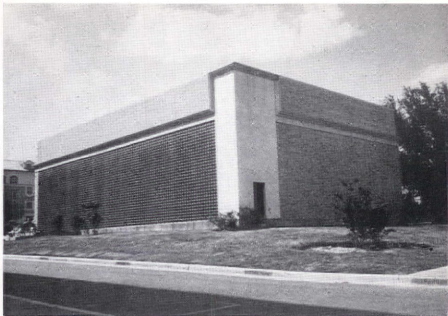
COOLING TOWER, CENTRAL AIR CONDITIONING PLANT, UNIVERSITY OF TEXAS, AUSTIN BROAD & NELSON, ARCHITECTS
