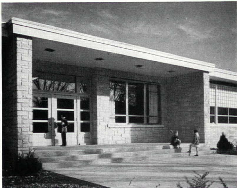
Elementary School, Western Springs, Illinois Photo courtesy American Air Filter Corp.
