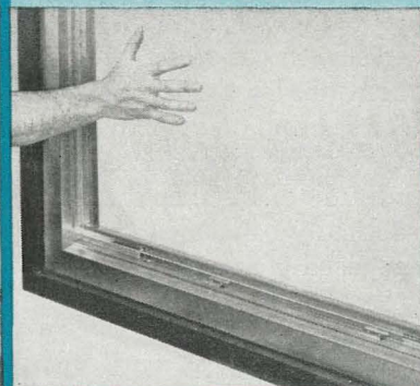
Place the glass on the setting blocks.
