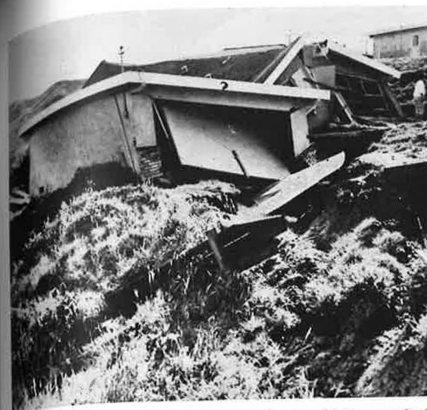
One of several homes in El Sobrante, Calif. wrecked by earthslides from heavy, drifting rains typical of hurricanes
