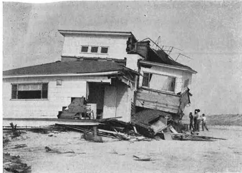
Beach property damaged and foundation completely undermined by battering wave wash (Long Island, N. Y.)
