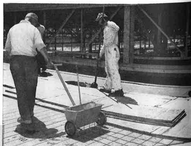
Fire protection without a vapor barrier! Where conditions do not require use of a vapor barrier, apply ribbons of adhesive to roof deck with the Lexsuco Spreader. Imbed insulation into ribbons of adhesive for dependable securement.
