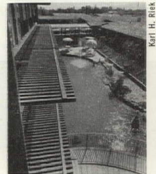
PLATE 14 Projected horizontal brise-soleil extends along the building at each floor level
