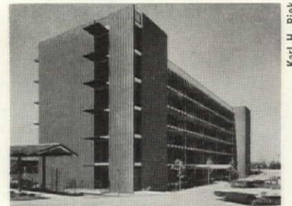
PLATE 13 Vertical grooved batten-lined forms at ends of building are painted to match the redwood
