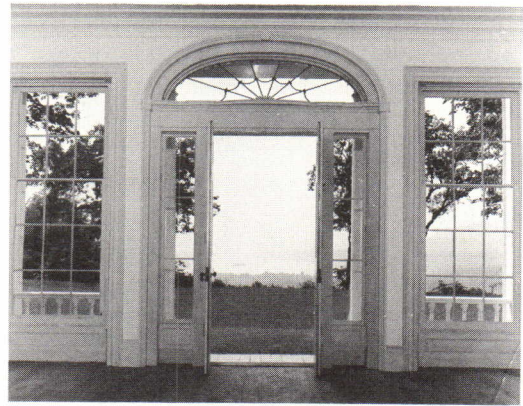
Main entrance doorway—interior view
