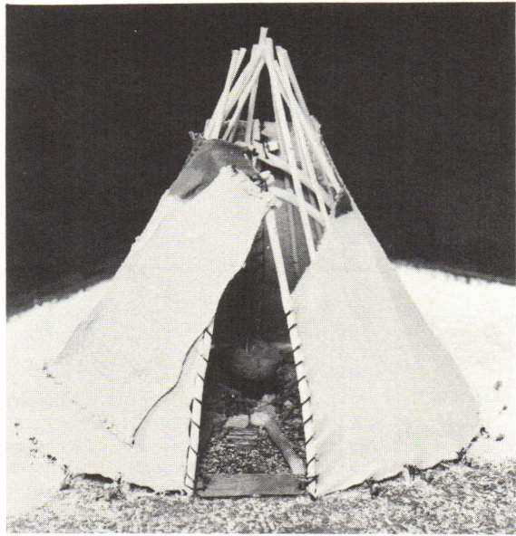
The Goatte, portable shelter of the nomadic Laplander, built of twelve to sixteen slender poles set around a curved frame of birch. A covering of reindeer hide or cloth is attached, leaving a four-foot smoke hole in the center above a ring of stones which forms the hearth
