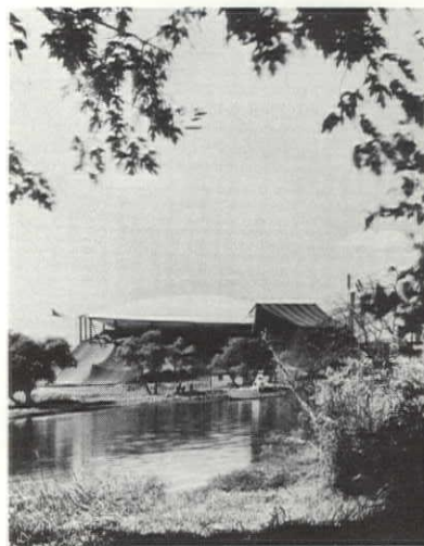
21 (Above) Five-cornered flat double membrane with center opening, border ropes. 22 (Below) In collaboration with Bird and engineer Paul Weidlinger, Carl Koch, AIA and Margret Ross roofed large open-air theater with nylon cushion
