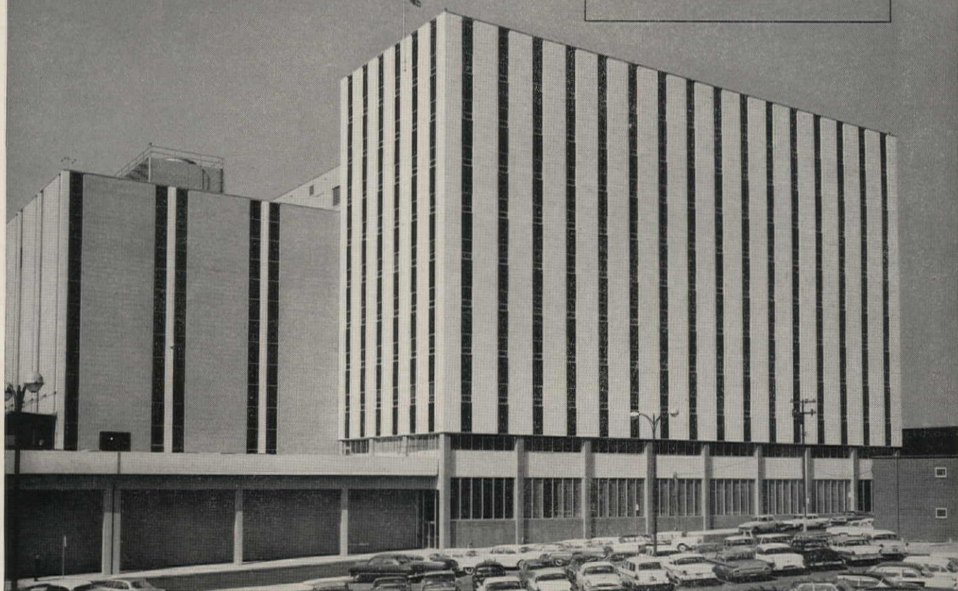
UNITED STATES POST OFFICE, DETROIT, MICHIGAN. Giffels and Rossetti— Architects-Engineers ; Barton-Malow Company— General Contractors . Administration Building and Mail Handling Building are faced with white textured Ceramic Veneer in unit sizes 5½" x 5½", 11" x 11" and 24" x 24". Thickness is 1¼" and 2¼". Polychrome seal in nine colors is 5' in diameter.
