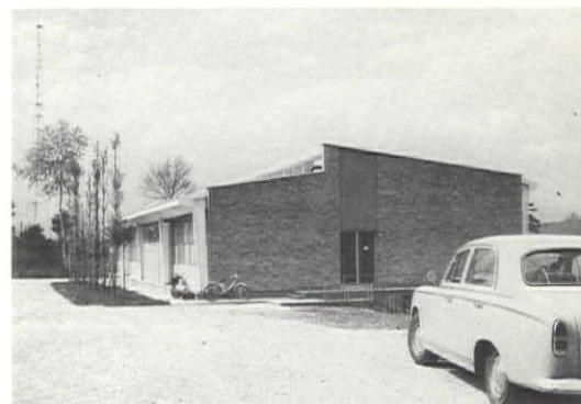
Laboratory, Ispra Reactor Center, Italy. Carlo Rusconi-Clerici, architect
