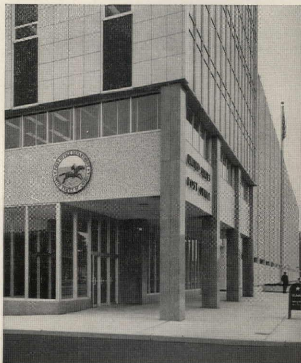
UNITED STATES POST OFFICE, DETROIT, MICHIGAN. Giffels and Rossetti— Architects-Engineers ; Barton-Malow Company— General Contractors . Administration Building and Mail Handling Building are faced with white textured Ceramic Veneer in unit sizes 5½" x 5½", 11" x 11" and 24" x 24". Thickness is 1¼" and 2¼". Polychrome seal in nine colors is 5' in diameter.
