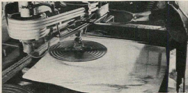
Sawn to thickness, then cut and shaped to 7' 11" at the wide points, each slab was hone finished on both sides to 1/4" and shipped, ready to install.
