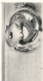
Amarlock long-throw bolt shows deeper penetration length. Chrome-plated steel sleeve is armored reinforcement.
