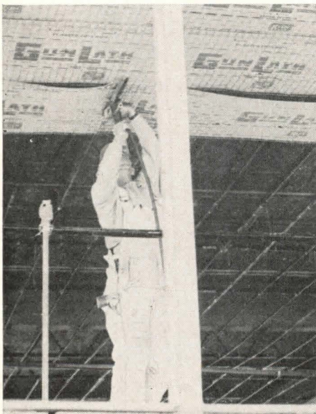
Mechanized lathing with K-LATH's GUN LATH.
