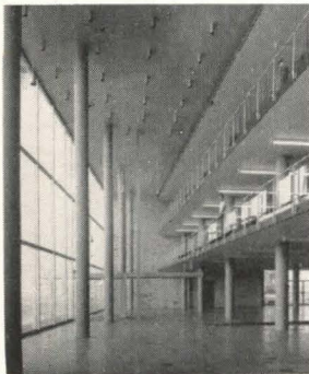
Dependable SONOTUBE Fibre Forms require minimum bracing and permit continuous pours as high as 40 feet.
