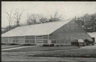
Municipal sewage treatment sludge bed
