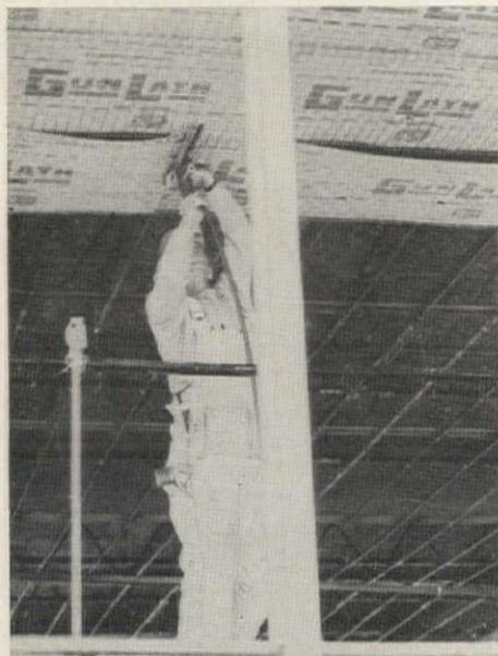
Mechanized lathing with K-LATH's GUN LATH.
